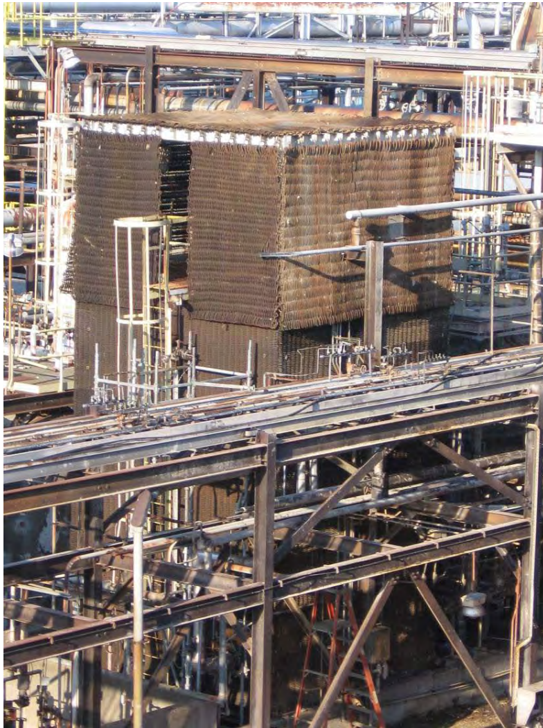
Figure 2. MIC day tank shield blanket structure
