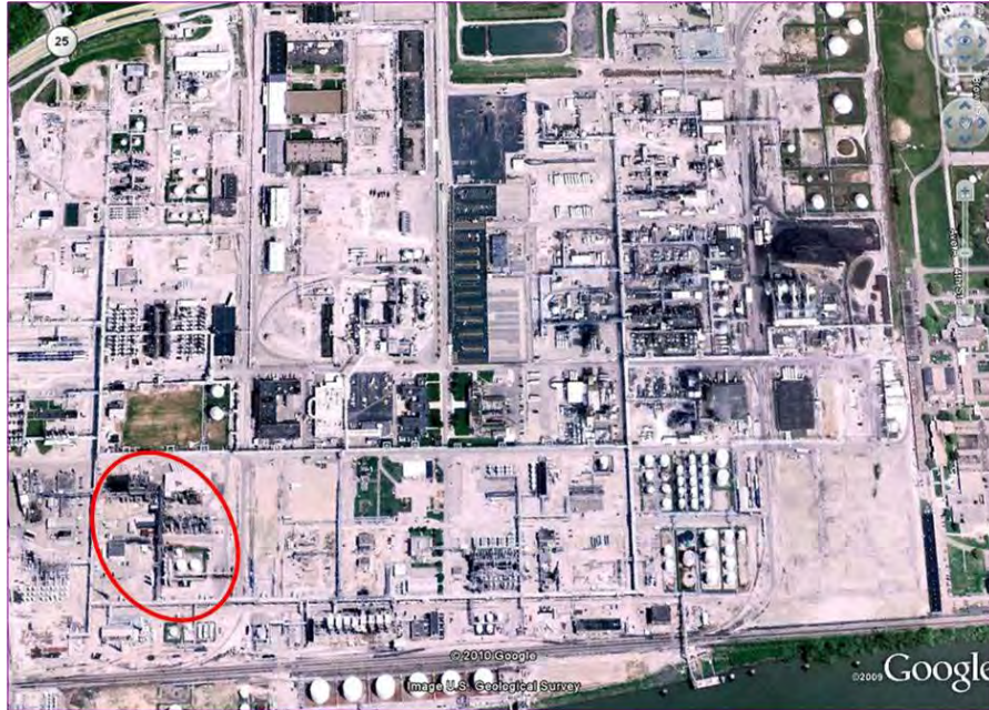
Figure 6. Aerial view of Bayer Institute Manufacturing Park. Methomyl-Larvin unit (circled) is in the West Carbamoylation Complex
