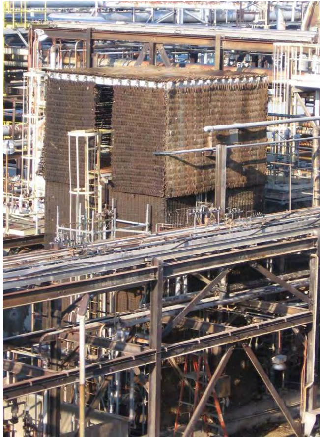
Figure C-2. MIC day tank shield structure
