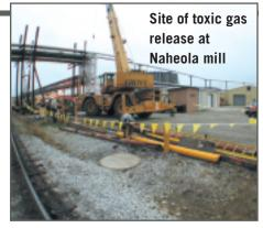
The hydrogen sulfide gas leaked through the seal of a fiberglass manhole cover near the Burkes construction workers. All ten victims were exposed to the escaping gas. Three workers were overcome almost immediately and fell to the ground. Instead of evacuating the area, three of the remaining workers attempted to drag the fallen men to fresh air. Two of them passed out in the course of assisting the others. Mill workers farther away saw the victims collapsing and called in emergency help.
