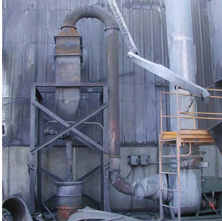
Figure 11. Fume separator and draft fan.
