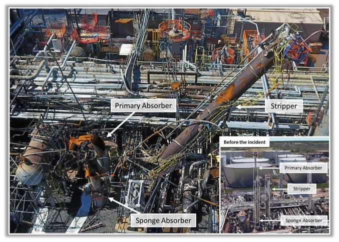
**Figure 44.** Primary absorber, sponge absorber, and stripper before and after the incident.<sup>a</sup> (Credit: Husky Superior Refinery and Google Earth with annotations by CSB)
