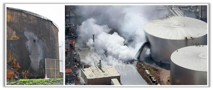
Figure 18. Asphalt tank puncture and leak. (Credit: CSB [left], Duluth News Tribune [right])
