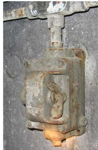
Figure 22. Non-dust rated and rated electrical devices in the silo tunnel
