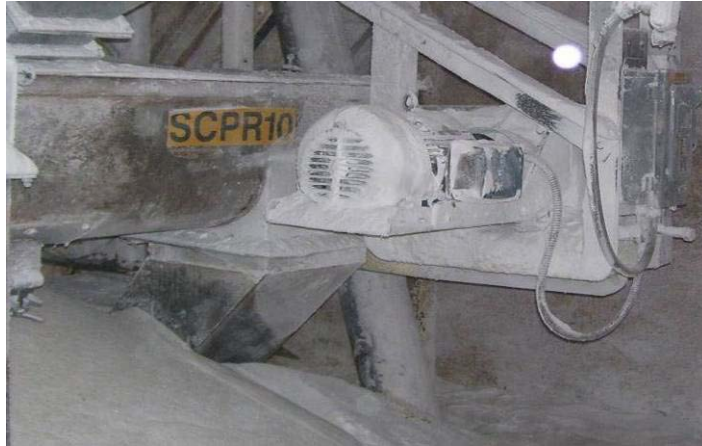
Figure 19. Motor cooling fins and fan guard covered with sugar dust; large piles of sugar cover the floor (Imperial Sugar photo)
