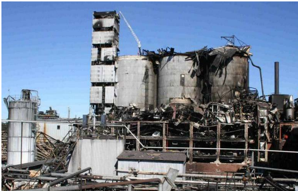
Figure 1. West bucket elevator tower; silos 3, 2, and 1; and south packing building destroyed by the February 7, 2008, sugar dust explosions and fires
