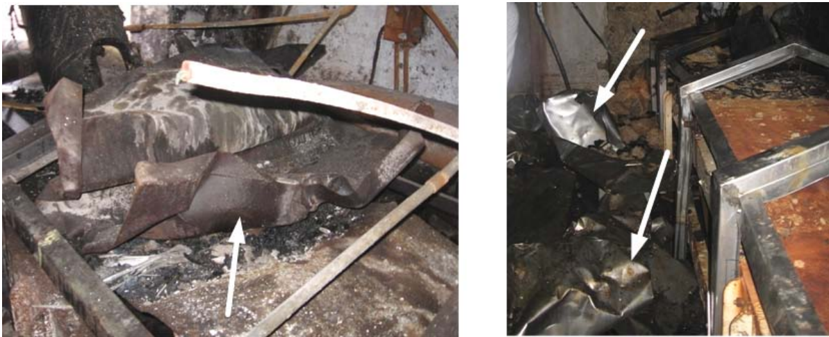
Figure 13. Steel belt covers (arrows) crumpled from an initial dust explosion inside the steel belt enclosure (steel frame structure, right photo)
