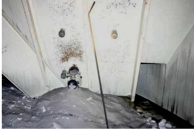
Figure 16. Access port inside the pantleg room and steel rod used to break sugar lumps in the sugar outlet on silo floor
