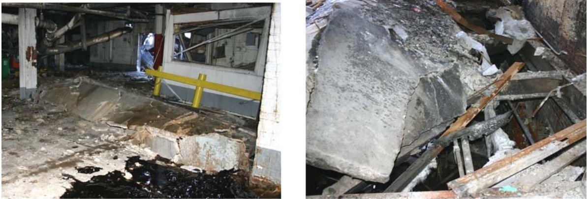
Figure 18. Three-inch thick concrete floor slabs lifted off the steel supports by the explosion pressure waves
