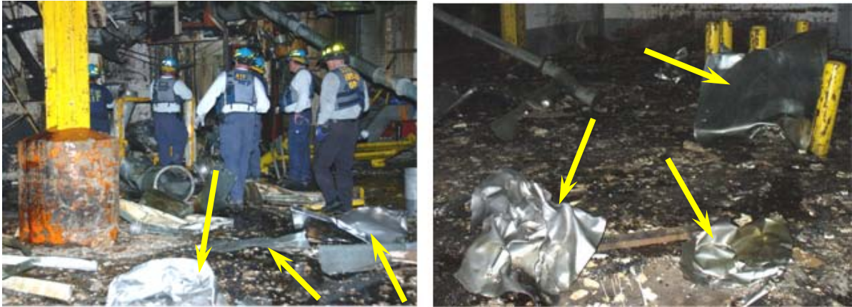
Figure 14. Stainless steel cover panels (arrows) blown off the steel belt enclosure and out of the tunnel into the packing building
