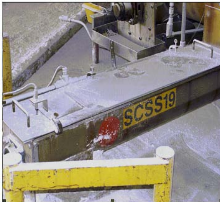
Figure 23. Sugar and dust accumulation on a screw conveyor in the south packing building fourth floor near silo 1 (Imperial Sugar photo)
