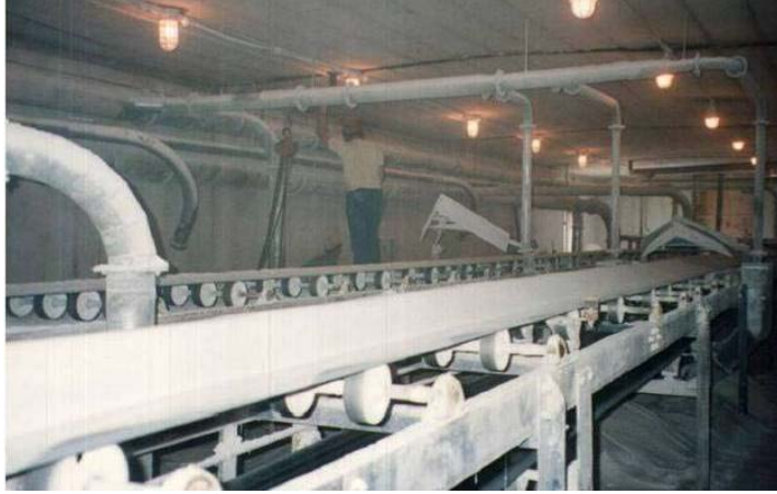
Figure 8. Granulated sugar steel conveyor belts above the silos, circa 1990. Heavy dust accumulation on conduit and spilled sugar on the floor (Imperial Sugar photo)
