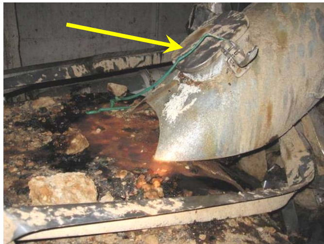
Figure 17. Limited clearance between sugar discharge chute and the steel belt would sometimes be blocked by large sugar lumps; lump-clearing access port (arrow) is on top of the chute
