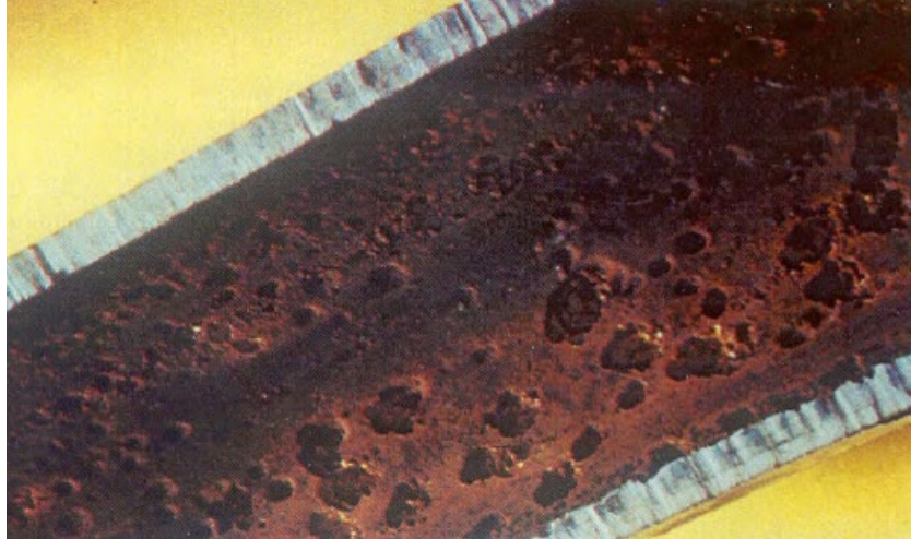
Figure 5. Pitting corrosion in a boiler tube. (Credit: U.S. Dept. of Defense [5, p. 38])
