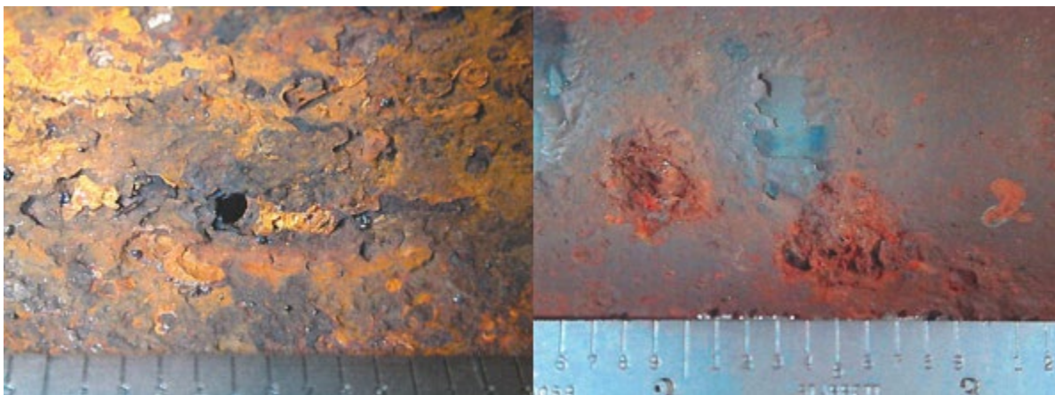
Figure 28. Pitting damage in two of Loy-Lange’s steam coils. (Credit: Clayton)
