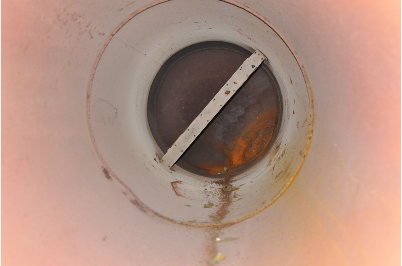
Figure 17. Photo of the inside surface of the SCR shell and upper head. (Credit: CSB)
