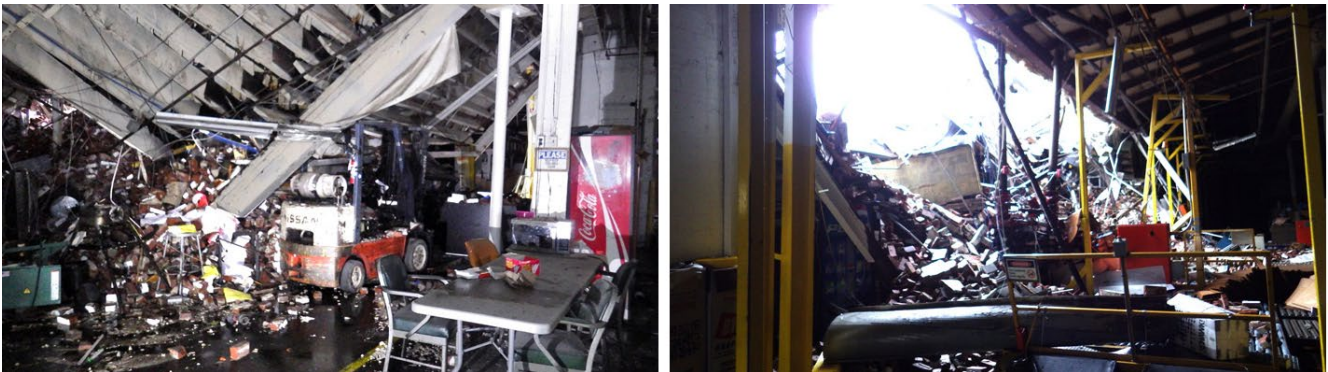
Figure 10. Photos of damage caused by SCR explosion. (Credit: St. Louis Fire Department)
