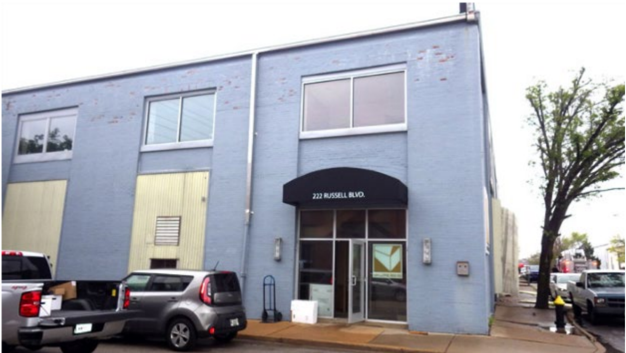
Figure 1. Loy-Lange Box Company, 1904 office building. (Credit: St. Louis Fire Department)
