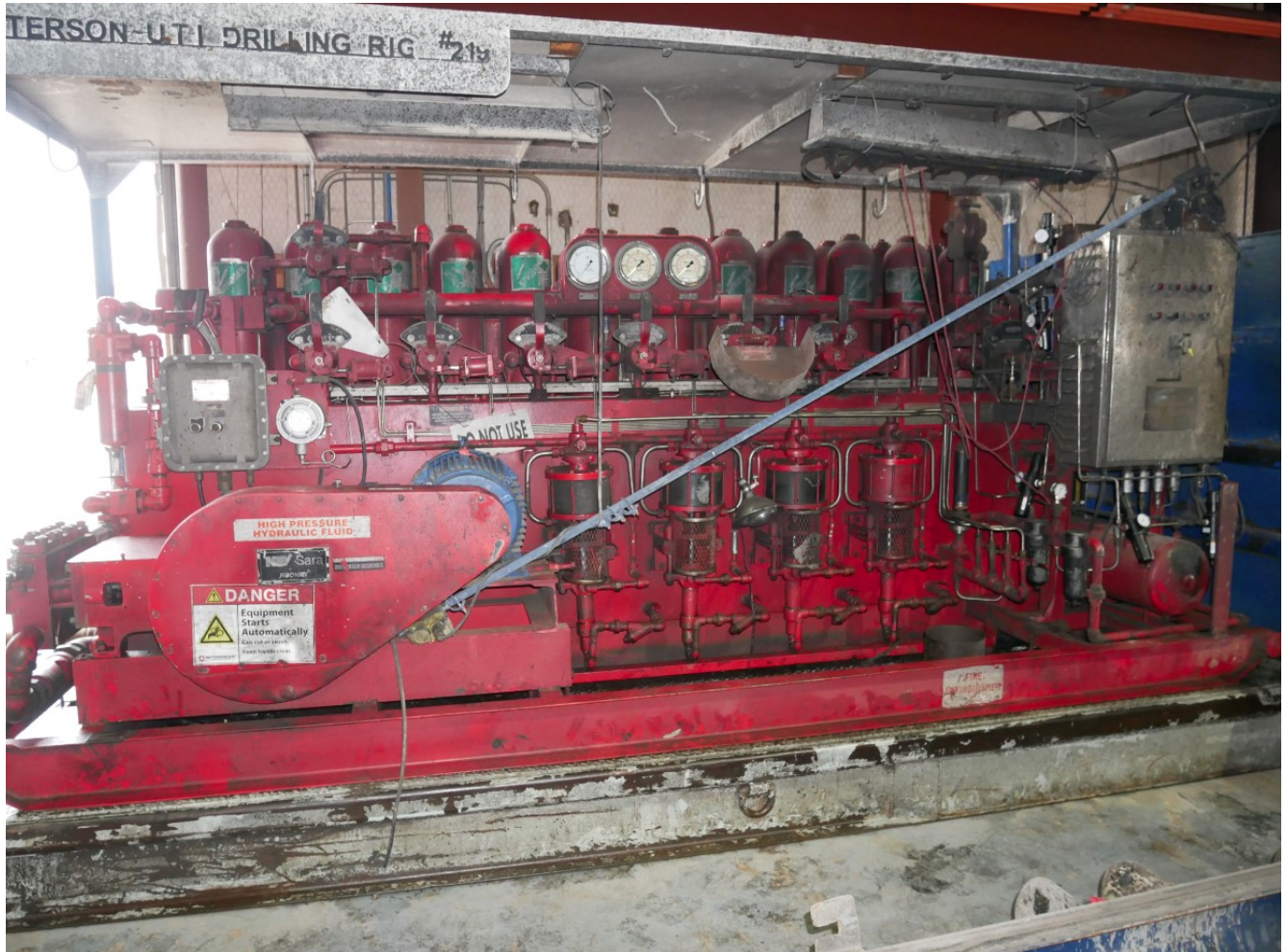
Figure A- 1. Photo of Patterson Rig 219 accumulator
