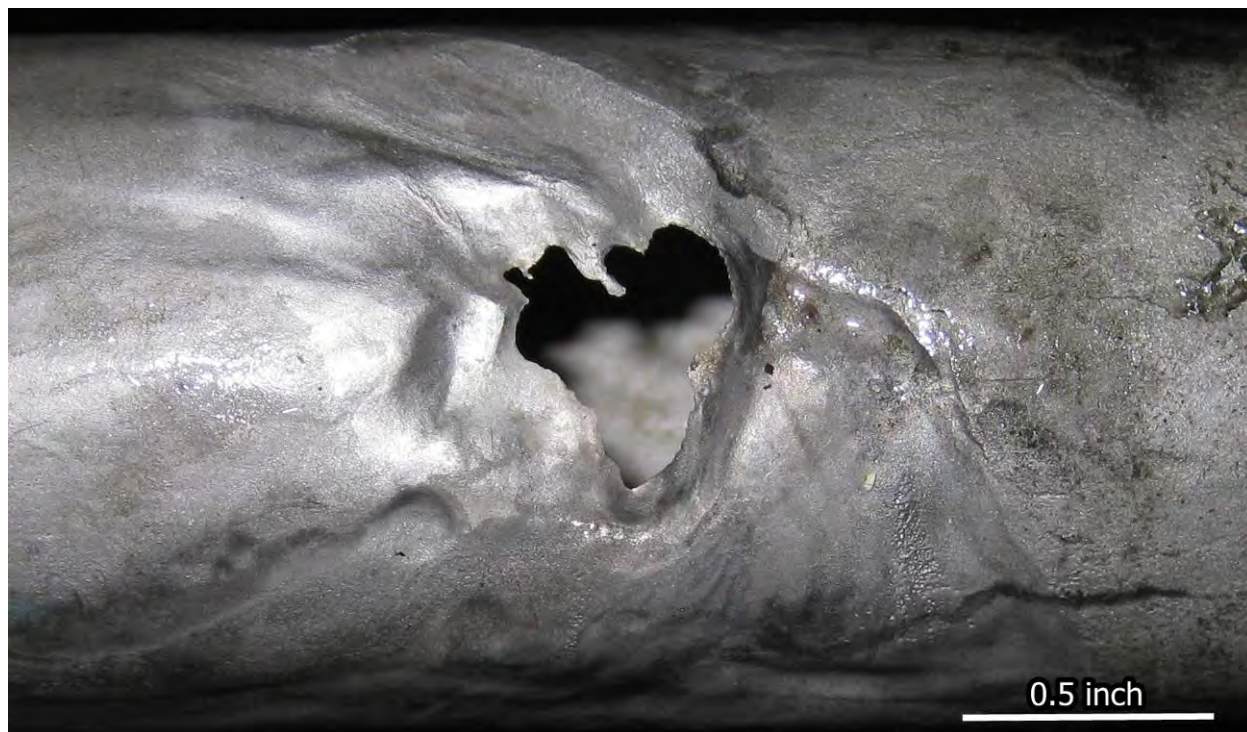
Figure 10. The large hole eroded from the outside-in on the oleum sample line 26
