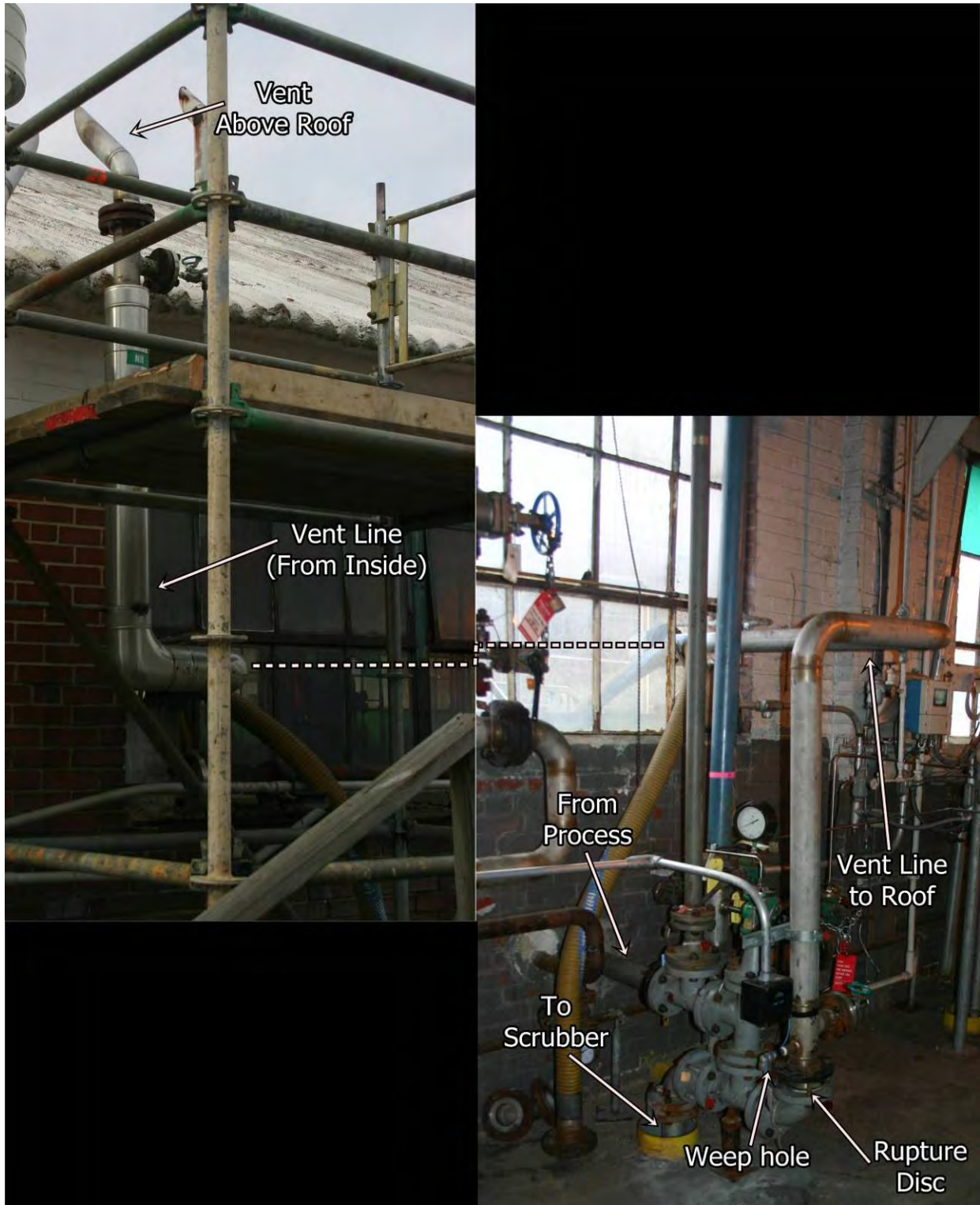
Figure 4. Rupture disc piping and vent pipeline to atmosphere on roof
