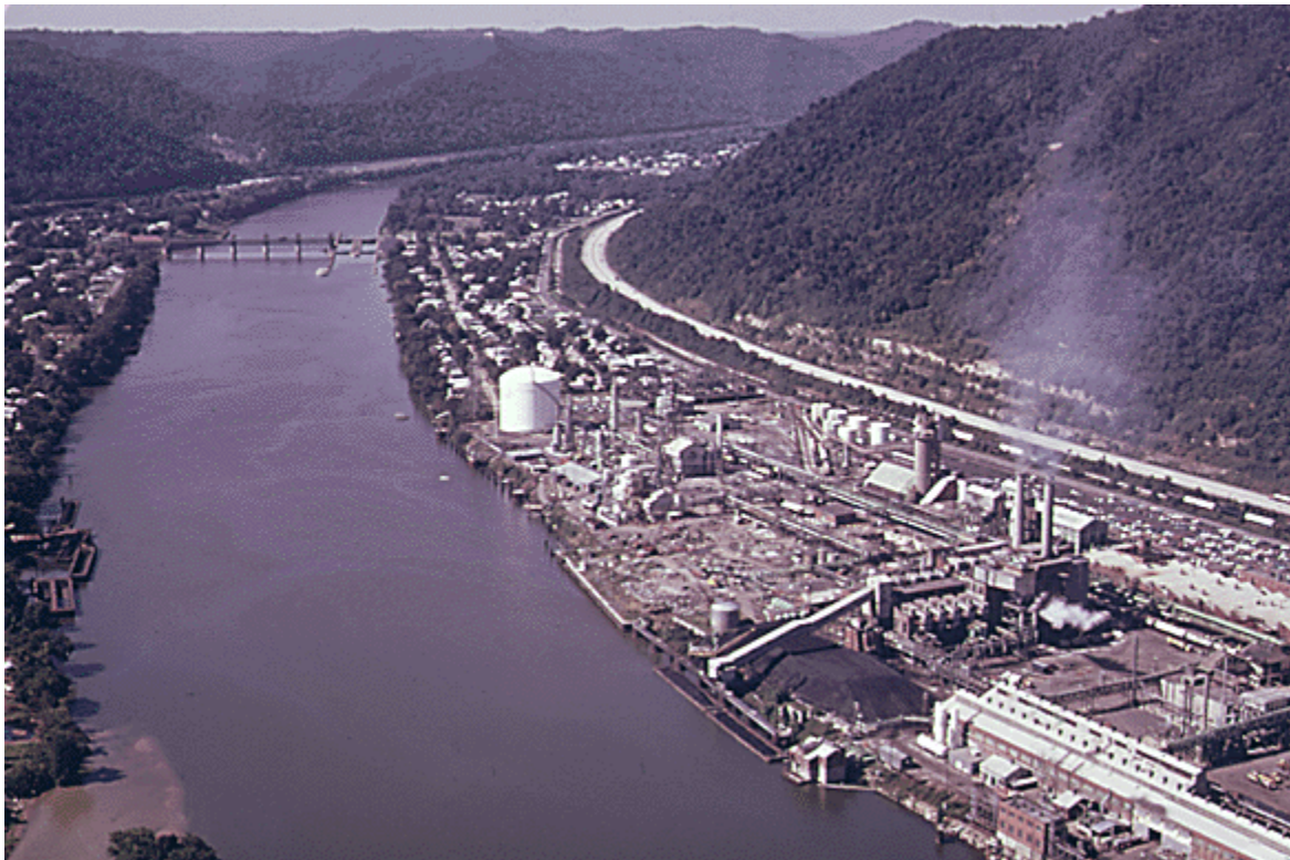
Figure 1. DuPont Belle, WV, facility on the Kanawha River (EPA, 1973)
