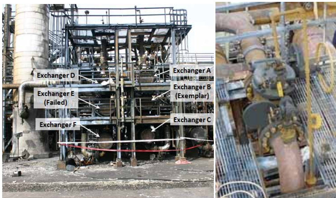
Figure 30. Unit structure (left) and manual block valve (right)
