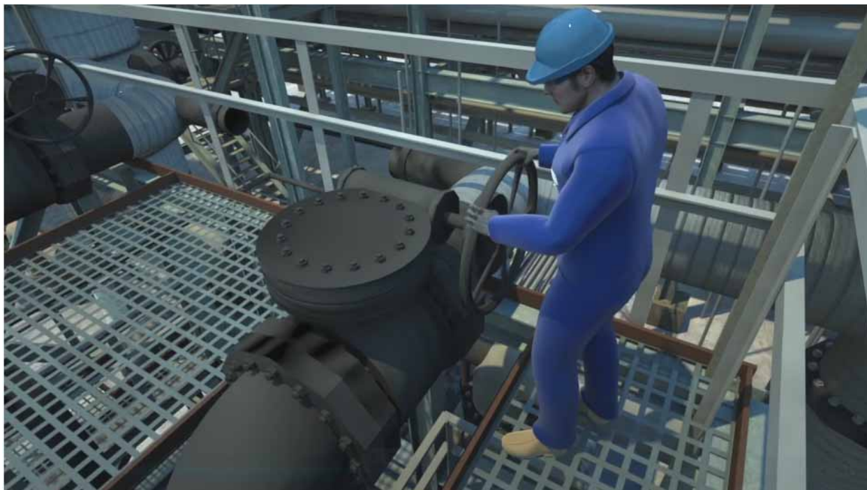
Figure 7. CSB Animation of Operator Opening Long-Winded Valve on Night of Incident. Valves on heat exchanger structure had to be opened concurrently when performing the heat exchanger bank startup
