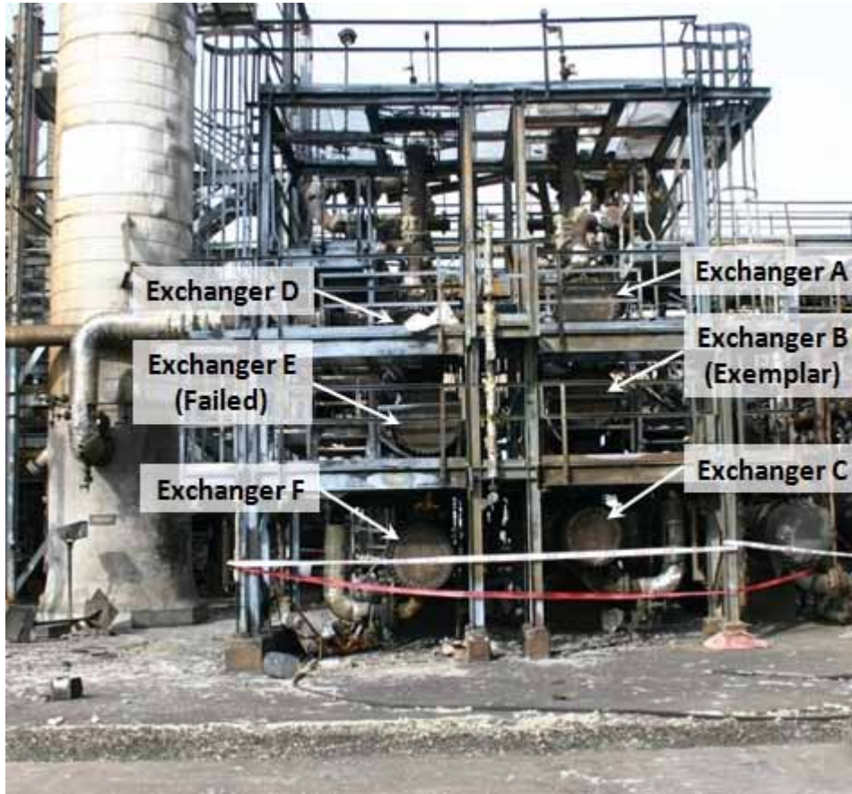
Figure 10. Six NHT Heat Exchangers in Two Banks of Three Heat Exchangers Each
