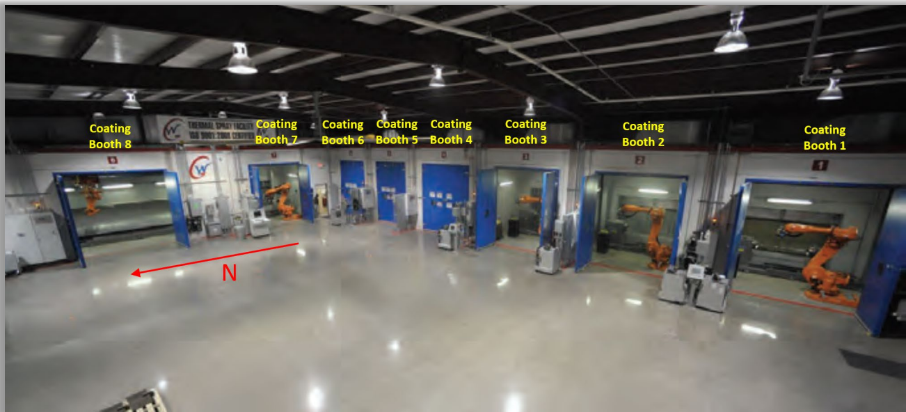
Figure 3. The Coating Building. The interior of the coating building was taken soon after construction was completed, circa 2010. (Source: Watson Grinding [3]; Annotations: CSB)
