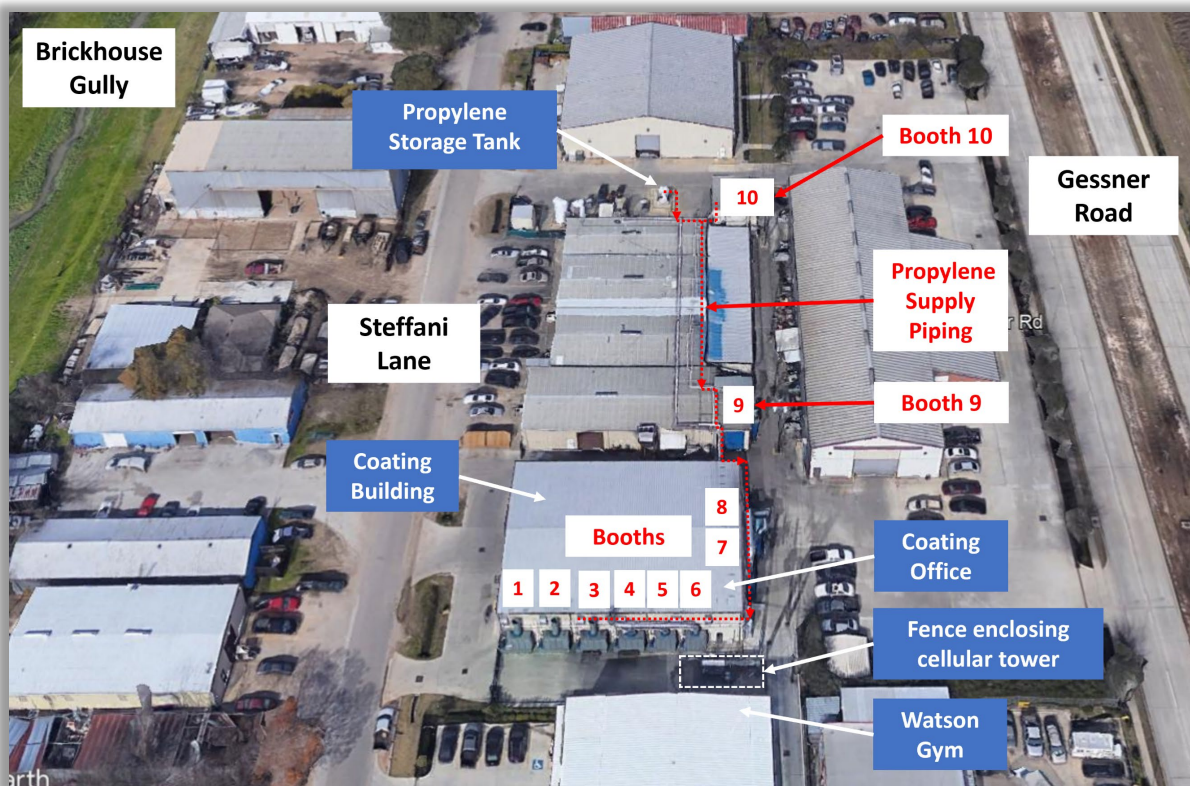
Figure 4. Propylene Supply Piping. This photo shows how Watson Grinding routed the propylene supply piping from the propylene storage tank to the eight HVOF coating booths. (Source: Google Earth Pro image from before the incident [7]; Annotations: CSB) d
