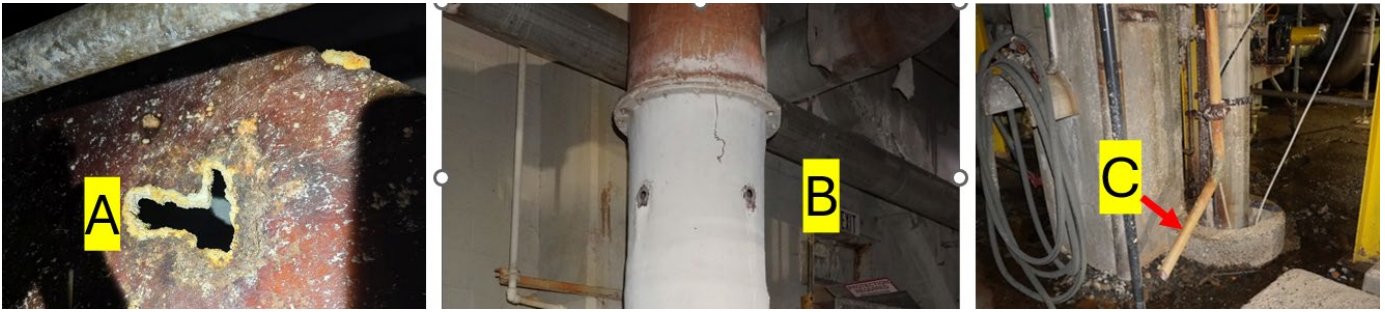
Figure 5. Process openings on the second floor of the Kraft Mill (Credit: CSB)
