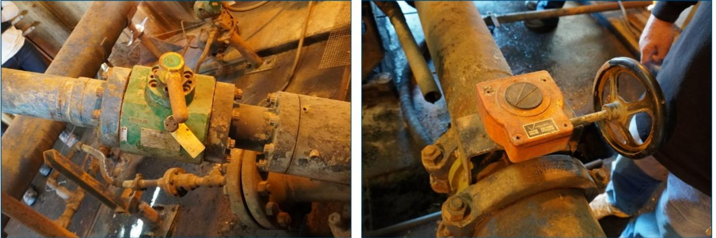
**Figure 19.** Position of the discharge (left) and suction (right) valves on Pump #1. (Credit: CSB)
