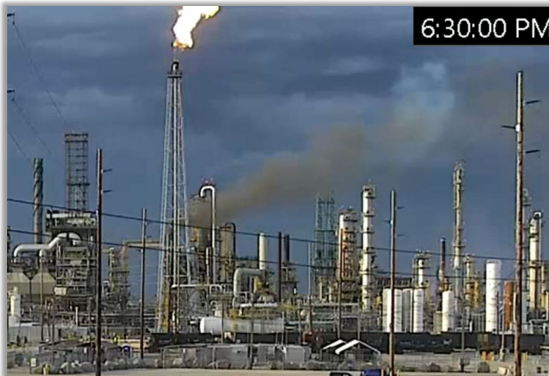
Figure 1. Smoking furnace and refinery flare prior to the incident. (Credit: BP)
