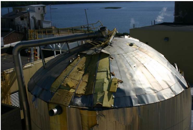
The CSB determined the explosion resulted from welding above an 80-foot-tall storage tank that contained highly flammable hydrogen gas – the product of bacterial decomposition of organic fiber waste inside the tank.
