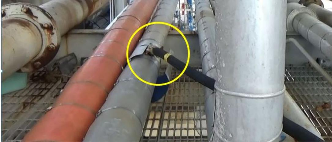
Figure 14. Hot water hose positioned on the liquid methyl mercaptan feed piping to flow hot water between the piping and the insulation in an effort to heat the piping and dissociate the solid hydrate that formed after water inadvertently entered the mercaptan storage tank.
