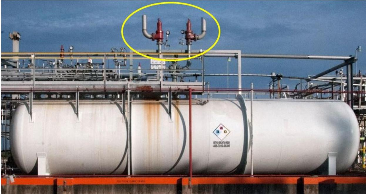
Figure 26. Methyl mercaptan storage tank showing atmospheric relief valves (yellow circle). At present, the storage tank is not insulated and there does not appear to be any mitigation to prevent off-site ERPG-3 concentrations as required by American Petroleum Institute and DuPont standards.
