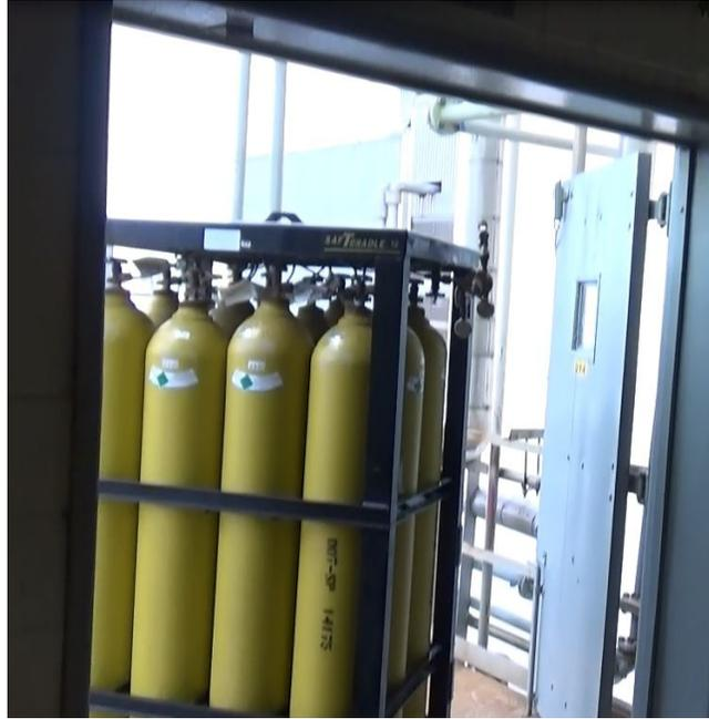
Figure 25. Photo of the open door on the south side of the second floor adversely impacting the dilution air ventilation flow across process equipment described in Figure 24.
