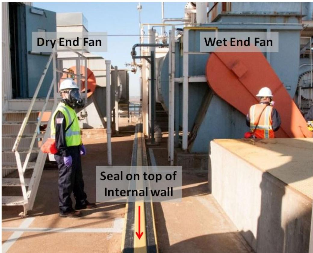
Figure 4. Roof of the manufacturing building showing the dry end fan (left), wet end fan (right), and location of the internal wall (middle) that separates each side within the building.
