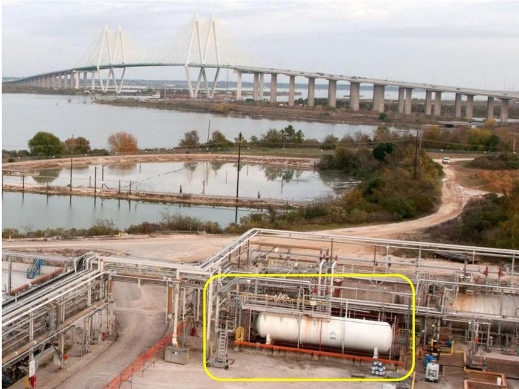
Figure 13. The yellow box outlines the 18,000 gallon methyl mercaptan storage tank at the DuPont facility in La Porte, Texas. Both the Lannate<sup>®</sup> and Vydate<sup>®</sup> insecticide processes use methyl mercaptan as a key raw material.
