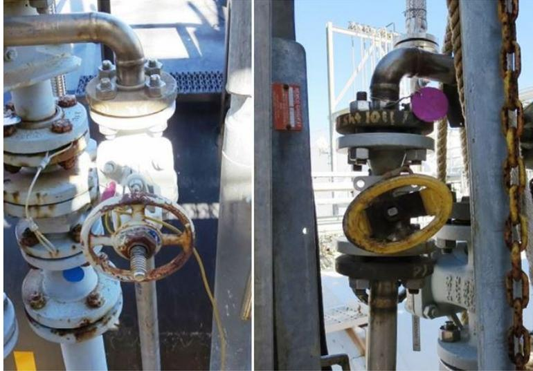
Figure 17. The fully open valve (left photo) and the cracked open valve (right photo) between the methyl mercaptan feed line and the waste gas vent header. These post-incident photos show the valve positions at the time of the incident.
