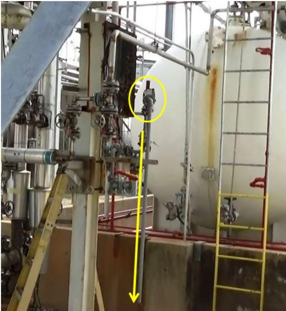
Figure 29. Liquid methyl mercaptan relief valve on the discharge of the methyl mercaptan pumps is designed to discharge this highly toxic, highly flammable chemical to grade just north of the methyl mercaptan storage tank.
