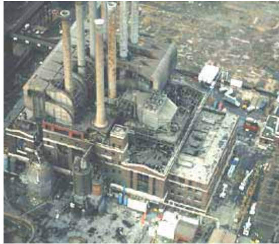
Figure 8. Aerial of the Ford River Rouge facility powerhouse. 19
