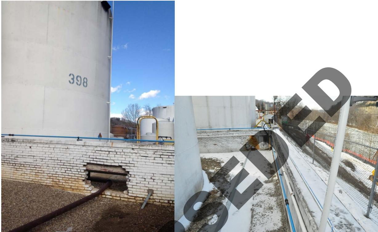
**Figure 24. The dike walls that surrounded the tank farms were in poor condition. (Source: CSB)**
