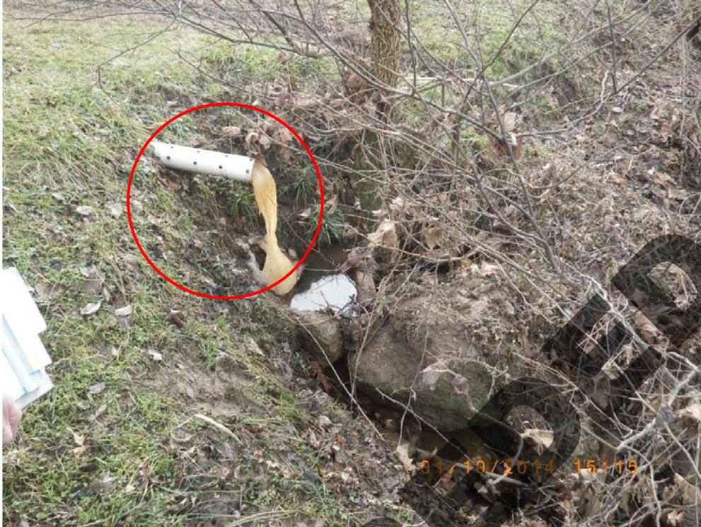
**Figure 25. Ice-filled oil/water separator discharge pipe into the Elk River. (Source: WVDEP)**
