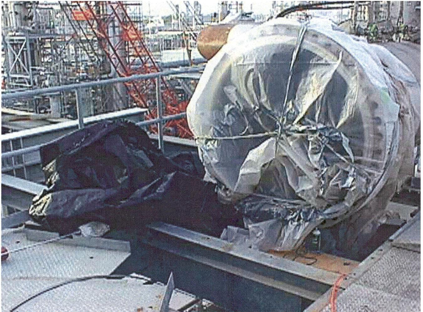
**Figure 2. Clear Plastic Sheet Covering One Of The Pipe Openings**
