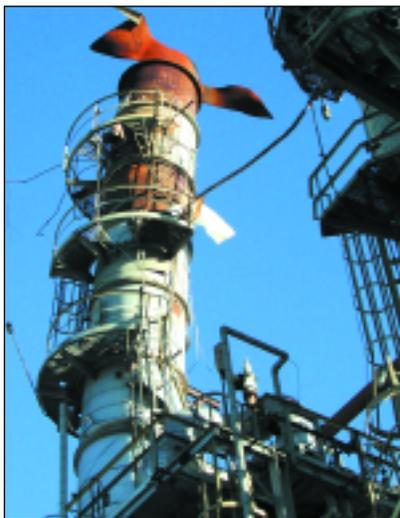
**Remnants of 145-foot distillation tower that exploded due to a violent chemical reaction.**
