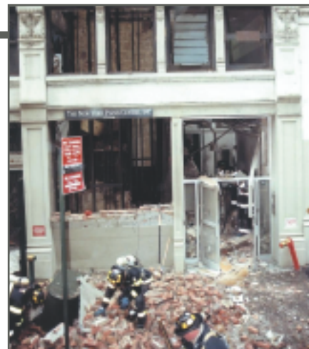
The explosion blew out windows up to the fifth floor and showered the street below with building debris.
