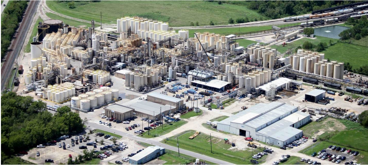
Figure 1. KMCO Facility in Crosby, Texas. a (Source: KMCO)
