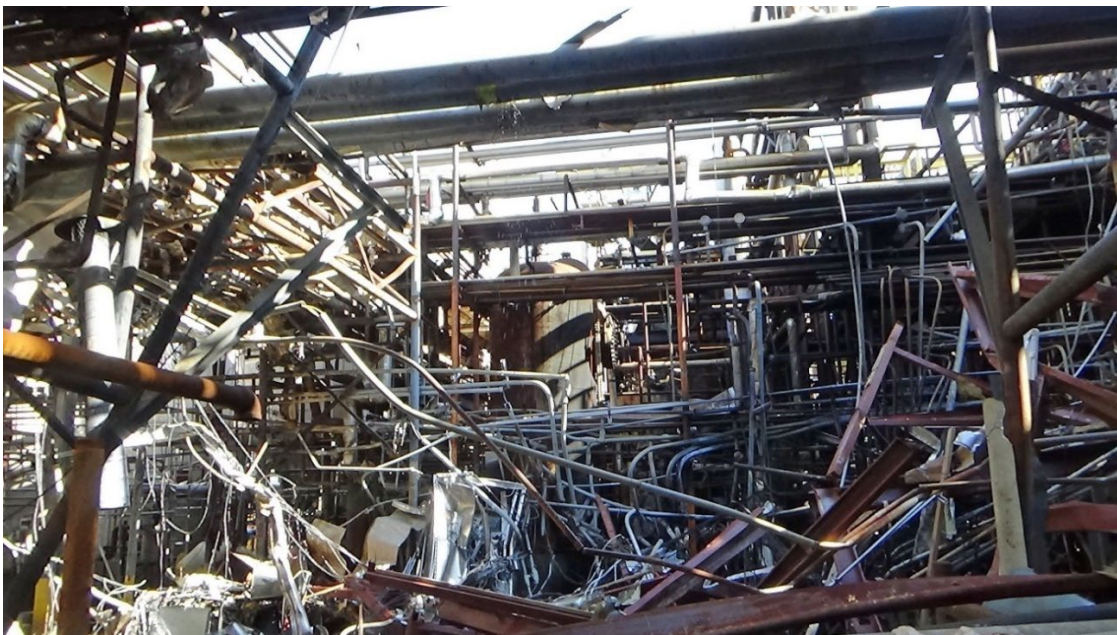
Figure 14. R2 Building (South Side). This post-incident photo shows the south side of the R2 Building. (Credit: CSB)
