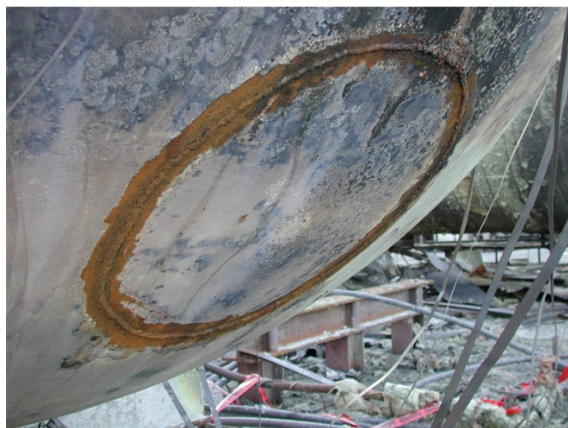
Figure 4. 24-inch patch plate on Tank 8.
