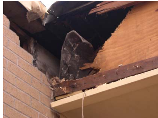
Figure 7. 20-pound Tank 7 fragment embedded in building wall 300 feet from the Marcus Oil property line.
