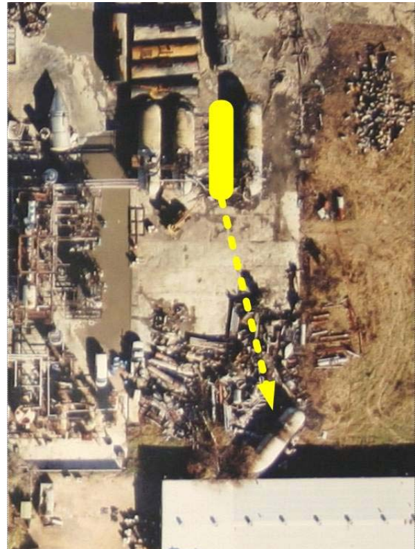
Figure 1. Explosion displaced Tank 7 more than 150 feet.
