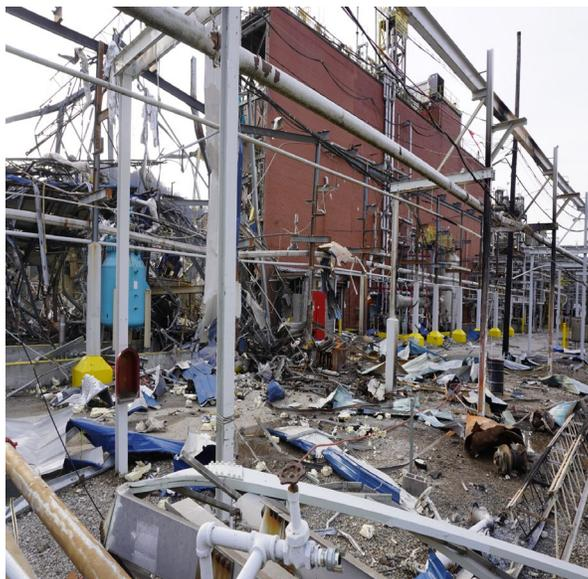
*Figure 1. Post-incident photo of the Optima Belle process building and area where the dryer unit was installed (Credit: CSB)*
