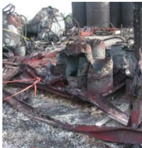
Figure 6. Drums located at packaging line 4.
