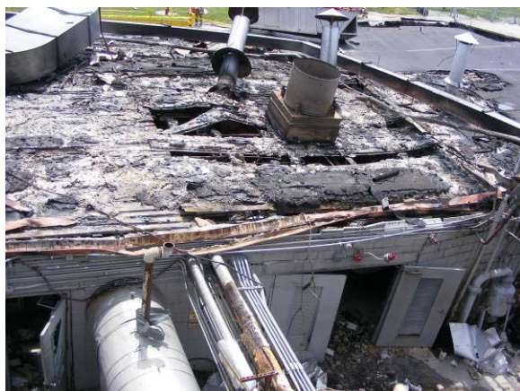
Figure 7. Roof and north wall of lab/operations building and boiler room
