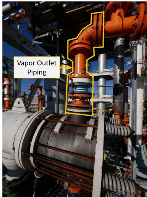
**Figure 2.** Jake Marshall Scope of Work. Wacker employees verbally requested the Jake Marshall employees check the torque on all of the bolts on the heat exchanger vapor outlet piping, which had been installed earlier in the week. (Credit: CSB)
