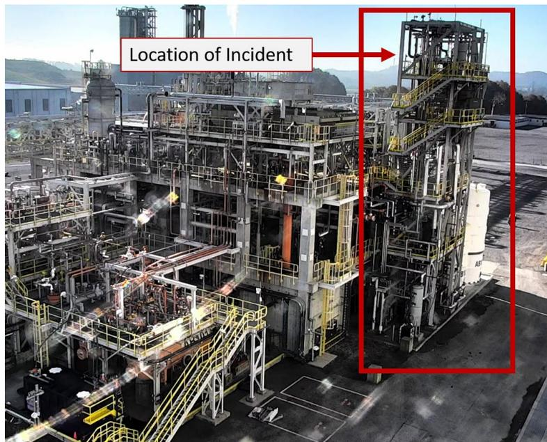
**Figure 1.** Five-story structure. The hydrogen chloride release occurred on the fifth floor of the structure. (Credit: Wacker)
