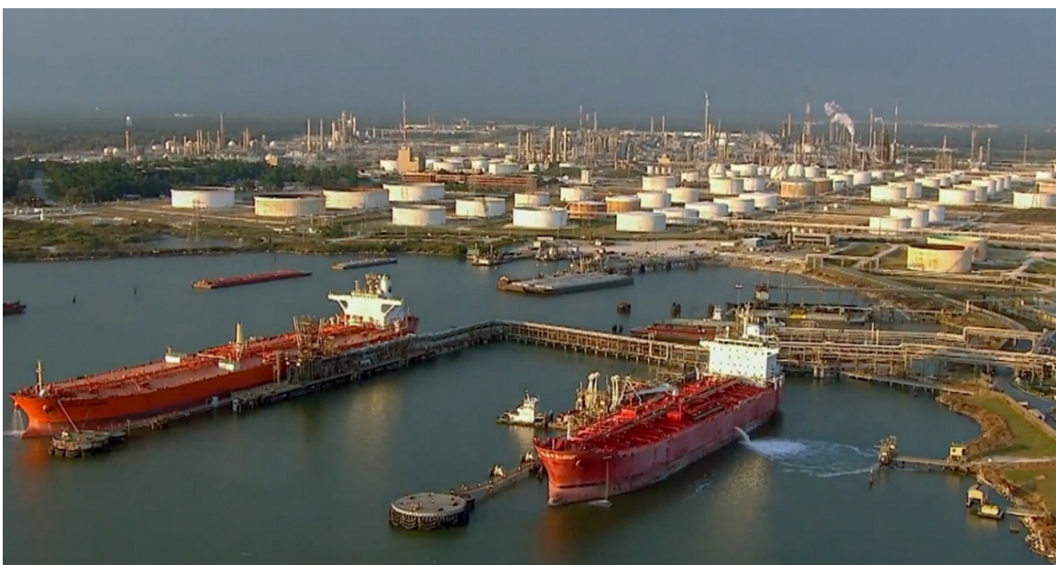
Figure 1. The ExxonMobil facility in Baytown, Texas. (Credit: CNBC)
