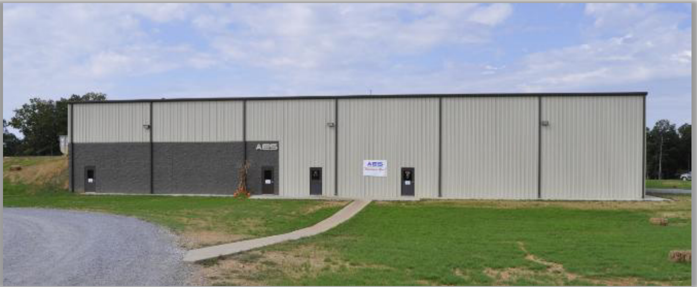
Figure 2. Pre-incident photo of Building 602. (Credit: AES)
