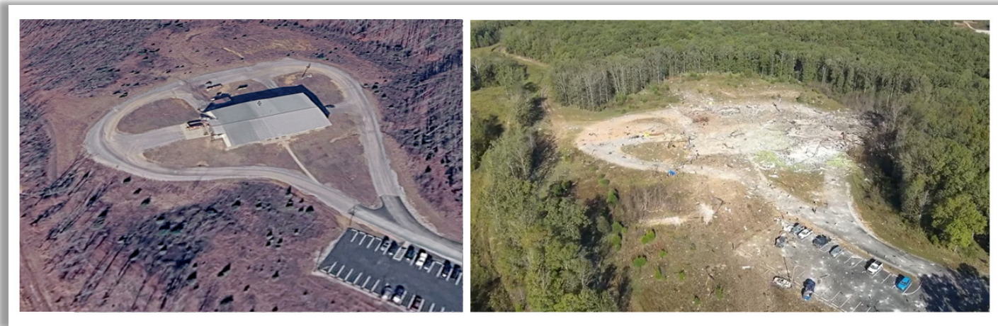
Figure 1. Incident building before (left) and after (right) the October 10, 2025, incident. (Credit: Google Earth (left); WZTV Nashville [2] (right))
