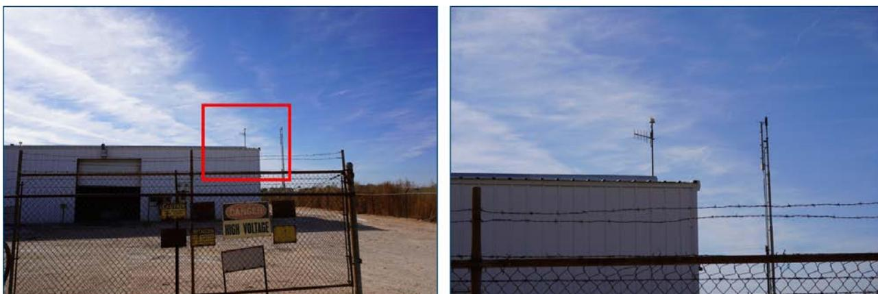
Figure 3. Light designed to illuminate when hydrogen sulfide is detected at the facility.
