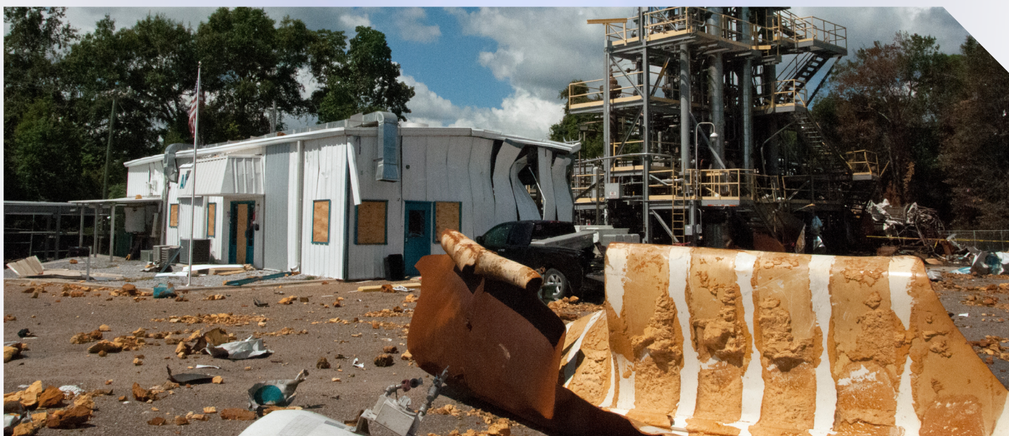
Post-incident photo of the administrative and operations building at the Airgas nitrous oxide manufacturing facility in Cantonment, Florida nitrous oxide manufacturing facility.
