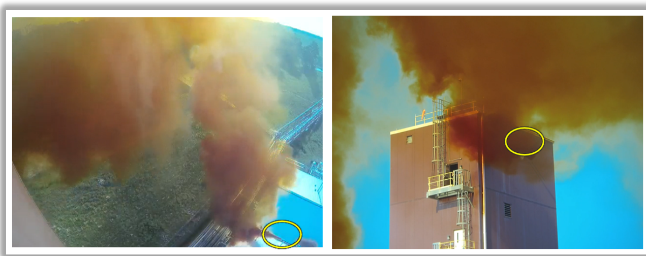
Figure 5. NO x release approximately one hour into the event (9:15 a.m.). The emergency pressure relief valve discharge (left) and absorber column vent (right) are circled. (Credit: Austin Powder, annotated by CSB)
