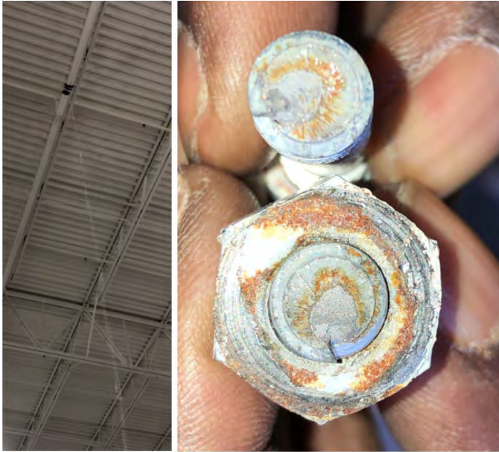
Figure 34. Failed fire protection piping coupling, pictured on December 30, 2019, due to bolt failure [left], and corroded cross-section of failed bolt [right]. (Credit: ARCO)
