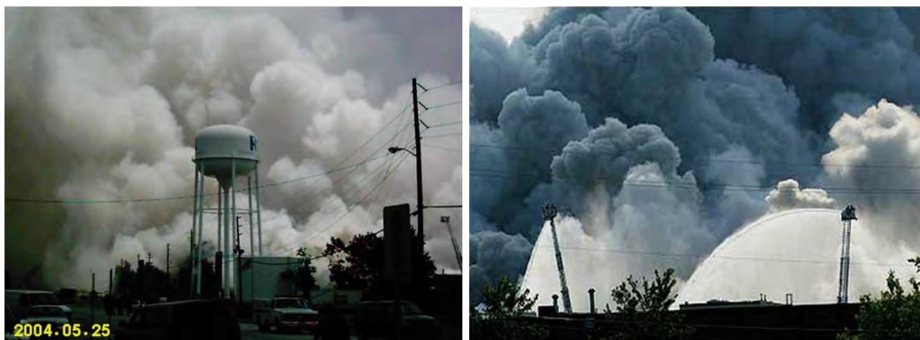
Figure 11. Chemical release and fire at Bio-Lab Conyers on May 25, 2004. (Credit: U.S. Environmental Protection Agency [29])
