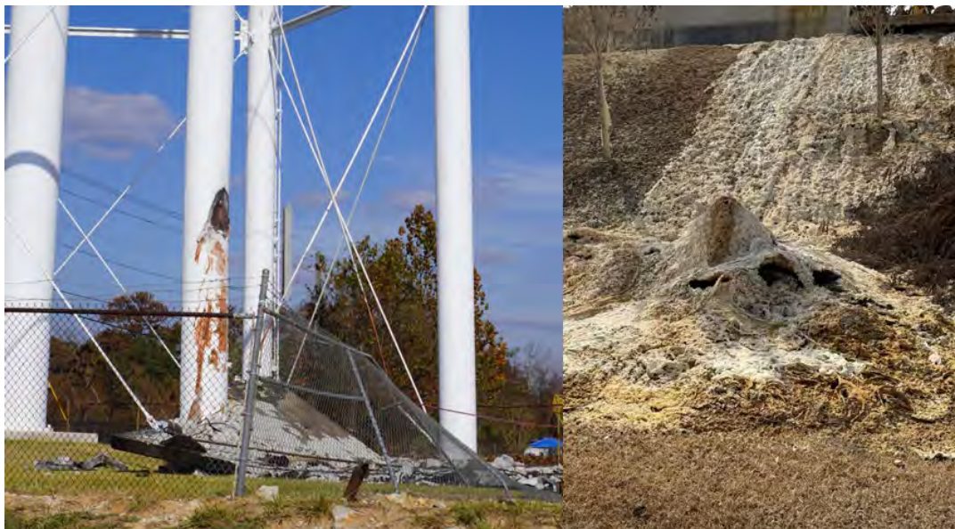
Figure 24. Damaged water tower supports struck by falling building walls (left) and reacting chemical material that spilled out after the bunker wall collapsed (right). (Credit: CSB [left], RCFR [right])
