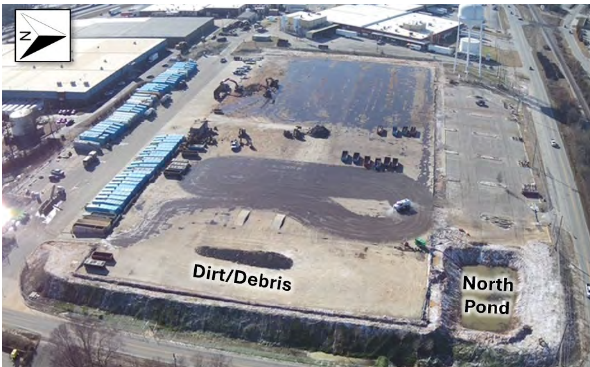
Figure 29. Concrete slab where the Plant 12 Storage Warehouse was located before the 2024 Bio-Lab Conyers incident. (Credit: KIK, annotated by CSB)
