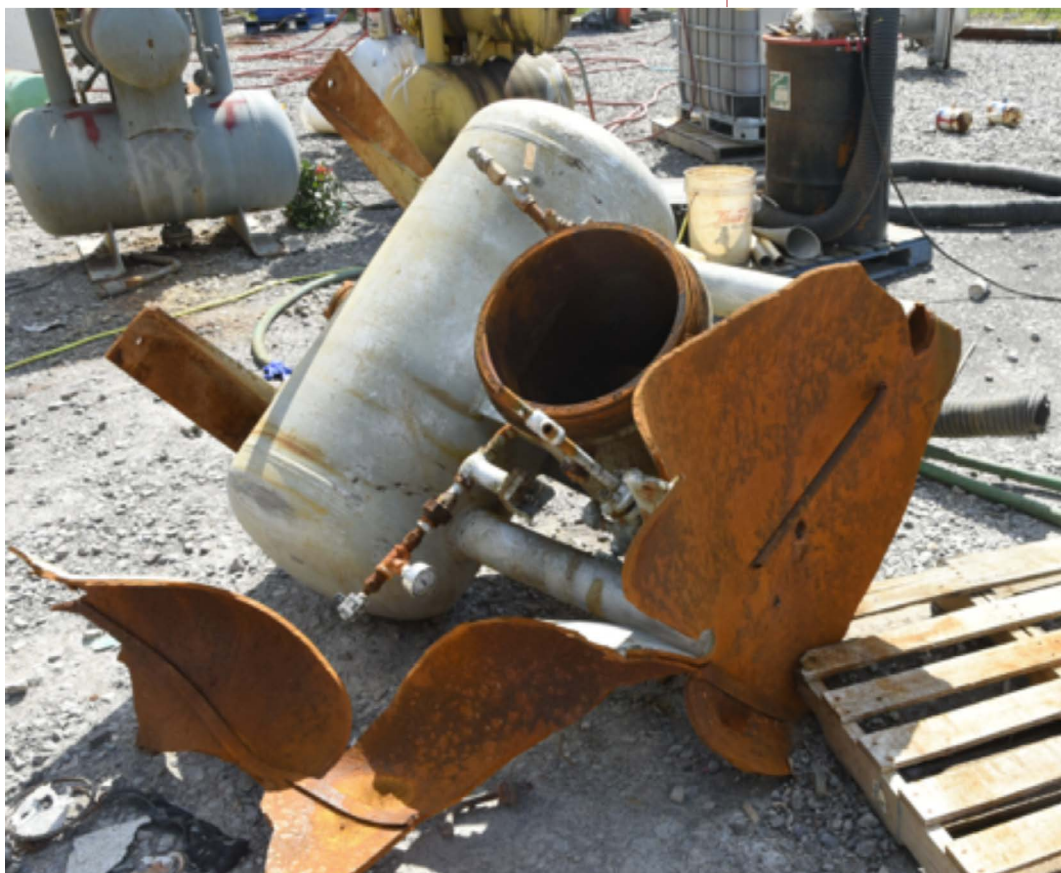
Figure 3. Tank that failed after the May 24, 2017 explosion. The middle tank failure was located at a threaded connection that connected an end cap to the middle tank.
