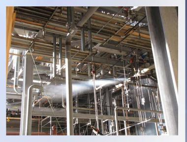
six and injured at least 50 people. The incident occurred while workers were conducting a "gas blow," where natural gas is forced through new piping and released into the atmosphere at a high pressure and volume in order to remove debris. As a part of its investigation, the CSB issued a recommendation to the Governor and Legislature of the State of Connecticut to enact legislation that prohibits gas blows. In September of 2010, the former Governor of Connecticut, M. Jodi Rell,
