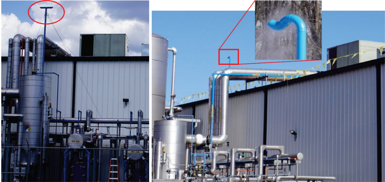
Figure 29: Tank Farm 5 atmospheric relief discharge piping, before (left, circled) and after (right, and inset) the incident. (Credit: CSB)
