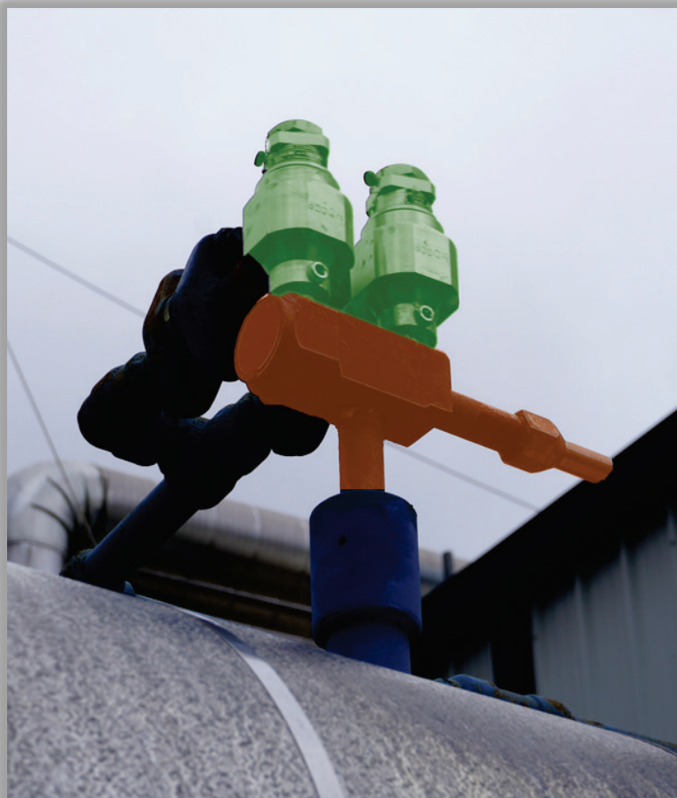
Figure 6: Emergency pressure relief valve assembly for a surge drum in Tank Farm 5, including two emergency pressure relief valves (green) and the three-way selector valve (orange). (Credit: CSB)
