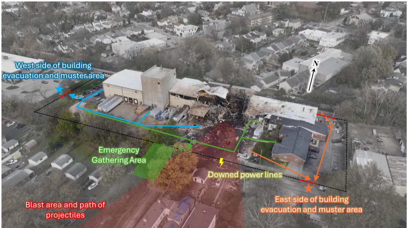
Figure 18. Depiction of the evacuation plan (green) versus the actual evacuation path taken by individuals at the facility (orange and blue). Personnel could not gather in emergency gathering area due to blast debris and a downed power line. (Credit: WAVE [13], annotated by CSB)
