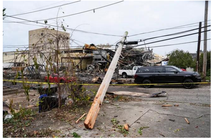
Figure 17. Damage to a nearby power line, which prevented employees from meeting at the planned muster location. (Credit: Matt Stone, Louisville Courier Journal [11])
