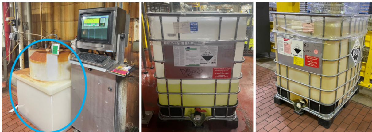
Figure 2. Photos showing the bleach solution tank (blue circle - left), a bleach solution tote (middle), and an acid solution tote (right). (Credit: Blues City Brewery, modified by the CSB)
