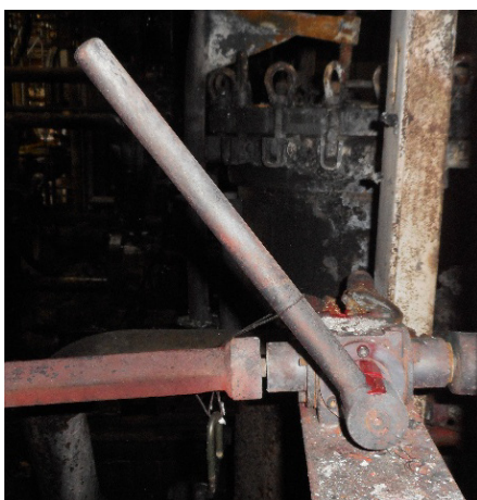
Figure 3. Locked out valve handle position. (Credit: Sasol)
