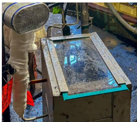
Figure 3. Enclosure installed after the incident. (Credit: Delek)
