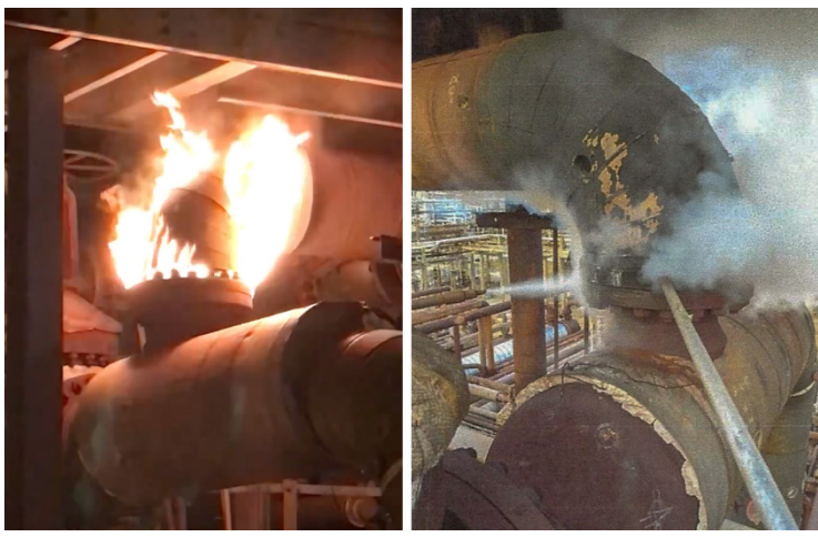
Figure 2. Fire on December 21, 2021 (left) and steam lances being used to keep the released naphtha from catching on fire (right). (Credit: ExxonMobil)
