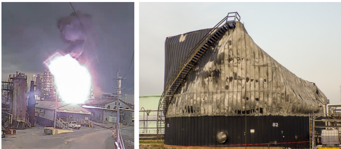
Figure 2. Tank explosion (left) and its post-incident condition (right). (Credit: Delek)
