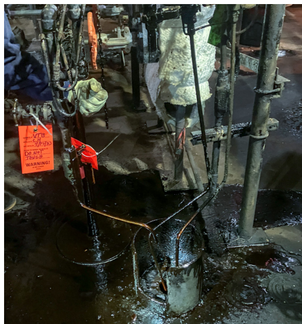
Figure 2. Post-incident image of the VTB release and sampling equipment. (Credit: Delek)
