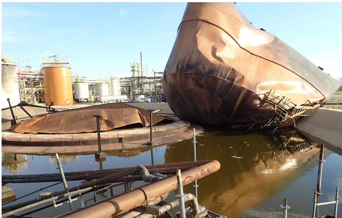
Figure 2. The tank after the explosion. (Credit: Westlake)
