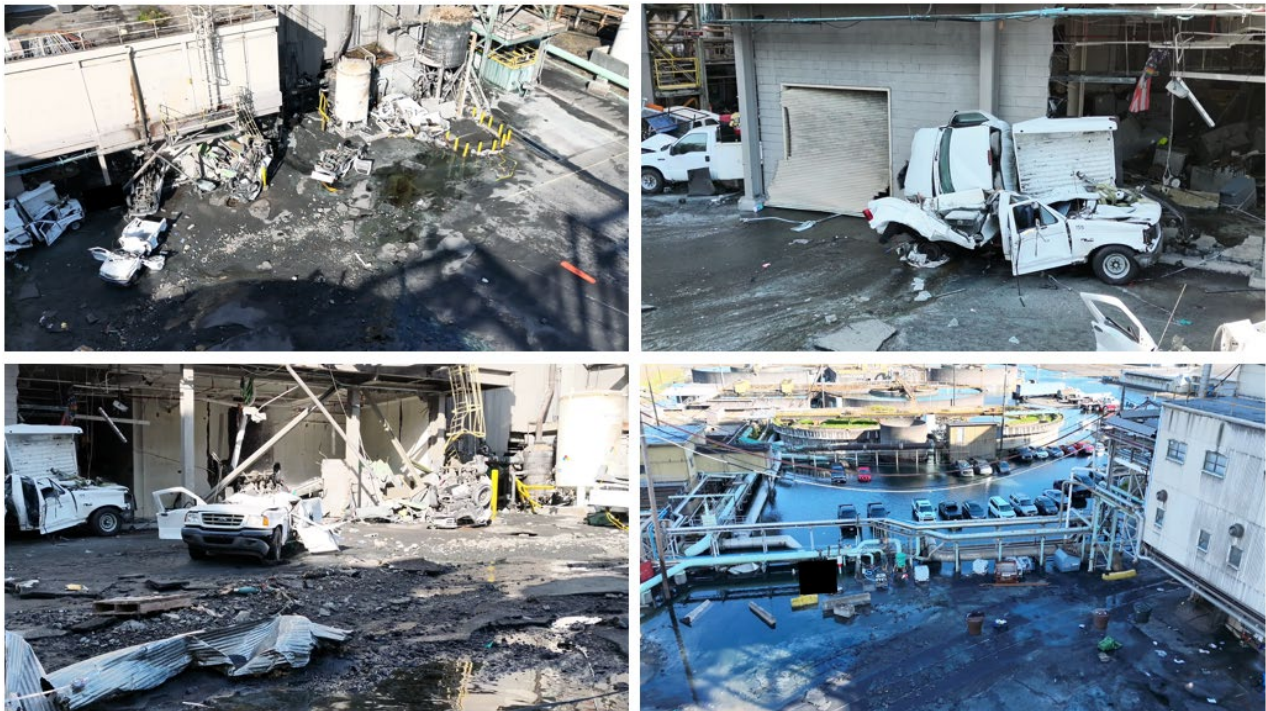
Figure 8. Damages from the G Tank failure. The images show the courtyard after the event, the crushed vehicles and damaged roll-up door, the destroyed wall, and a nearby flooded parking lot. (Credit Cowlitz County Sheriff, modified by CSB)
