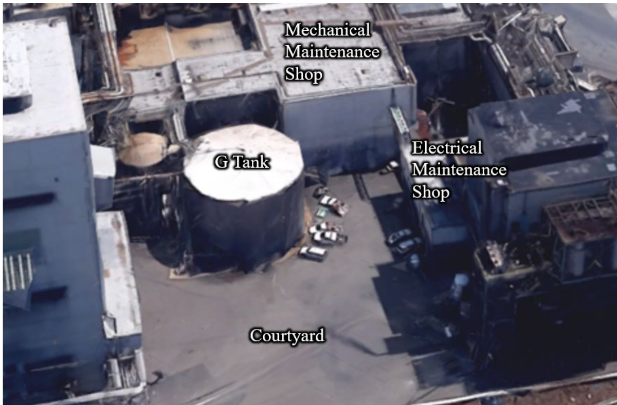
Figure 3. A pre-incident satellite image of the courtyard where G tank was built. (Credit: Google Earth, annotated by CSB)
