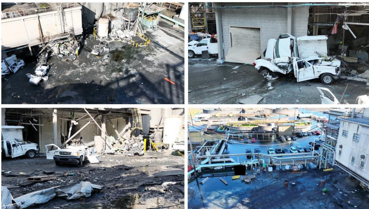
Figure 8. Damages from the G Tank failure. The images show the courtyard after the event, the crushed vehicles and damaged roll-up door, the destroyed wall, and a nearby flooded parking lot. (Credit Cowlitz County Sheriff, modified by CSB)
