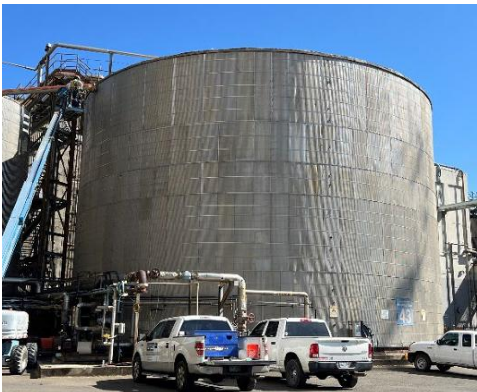
Figure 2. A pre-incident photo of G Tank. (Credit: NDP)
