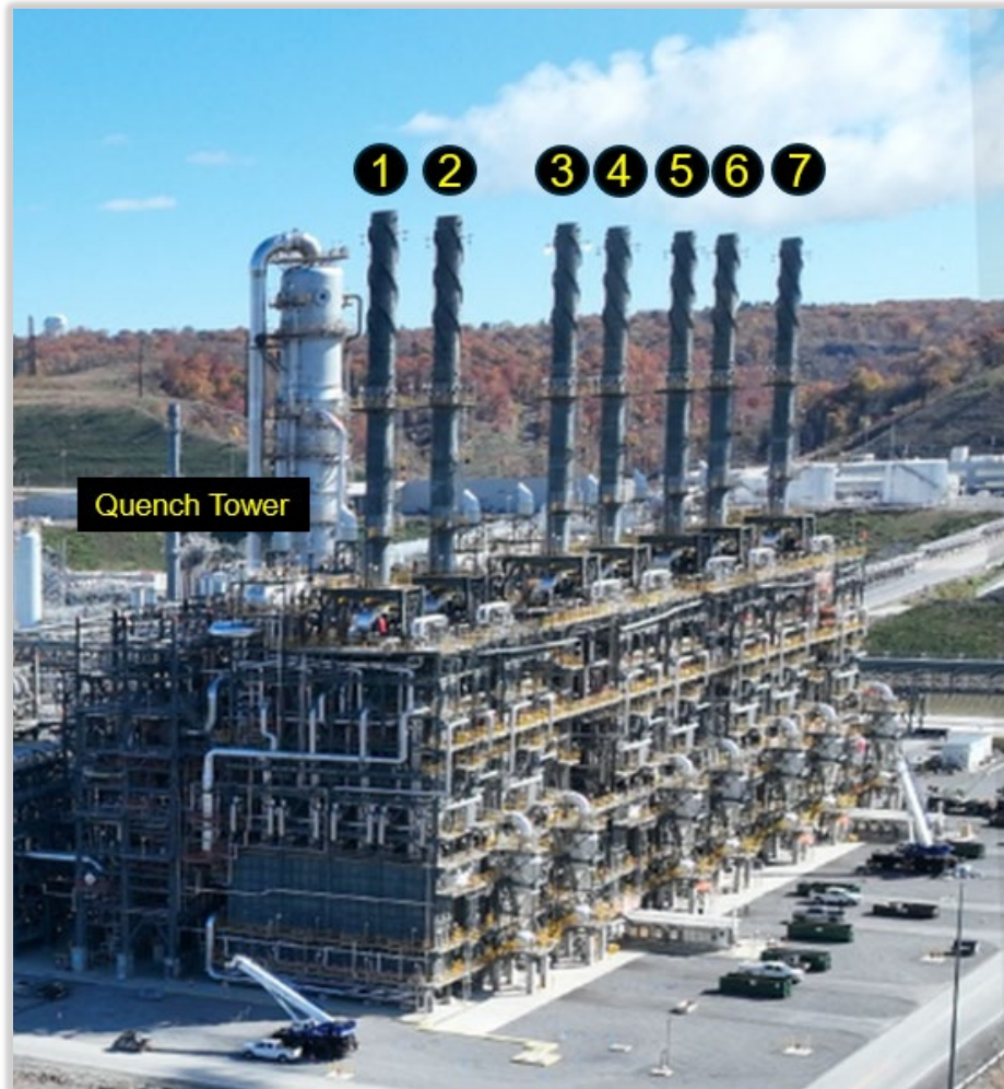
Figure 6. The seven ethane cracking furnaces and the quench tower at Shell Polymers Monaca. (Credit: Shell, annotated by CSB)
