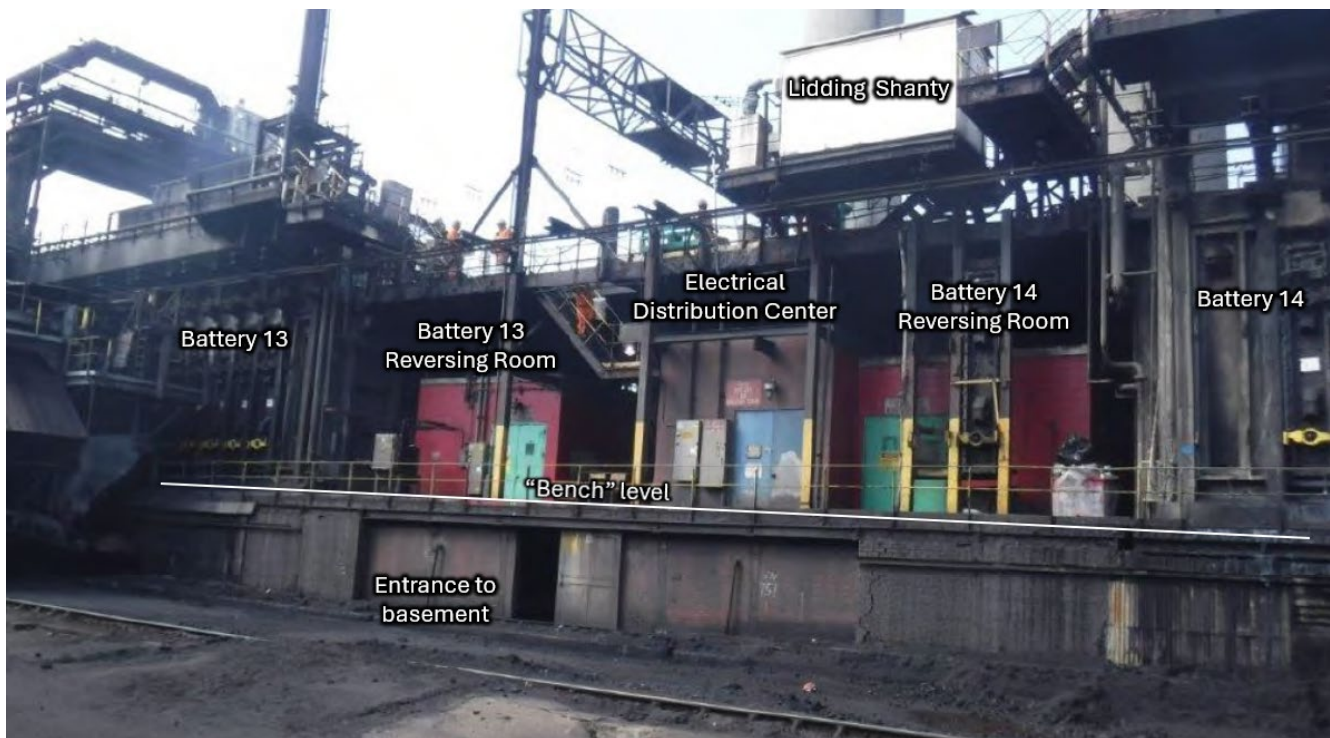
Figure 20. Pre-incident photo, date unknown, of the 13/14 transfer area. The break room is not pictured, as it was located behind the EDC and the Battery 14 reversing room. (Credit: U.S. Steel, annotated by CSB)
