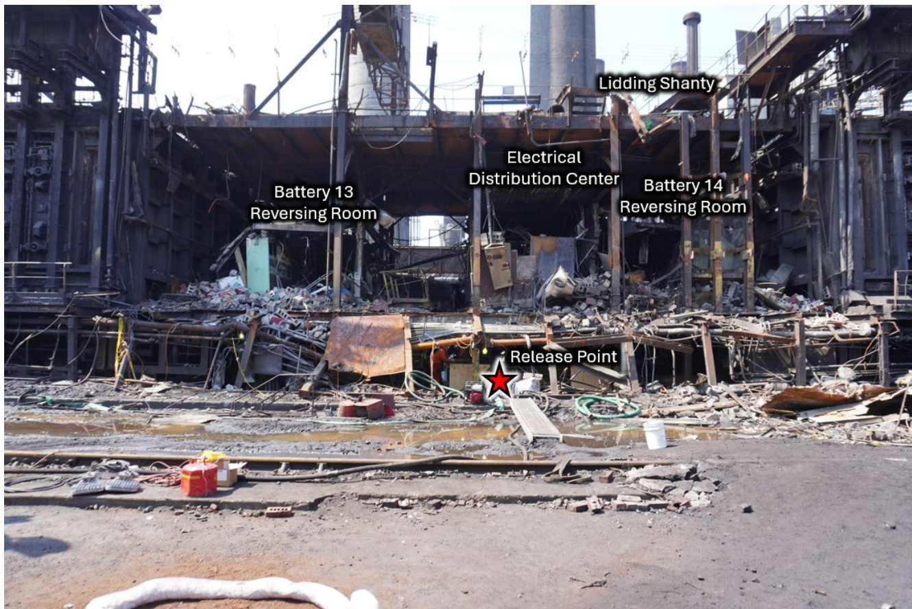
Figure 21. Post-incident photo of the 13/14 transfer area. The break room was located behind the EDC and the Battery 14 reversing room. (Credit: CSB)
