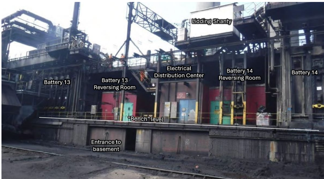
Figure 5. Pre-incident photo of the Battery 13/14 Transfer Area, showing the reversing rooms and other buildings. The break room is not pictured because it was located on the bench level behind the buildings shown here. (Credit: U.S. Steel, annotated by CSB)
