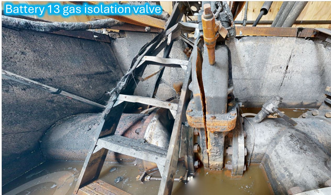
Figure 4. Battery 13 gas isolation valve as found post-incident (Credit: Allegheny County Fire Marshall, annotated by CSB)
