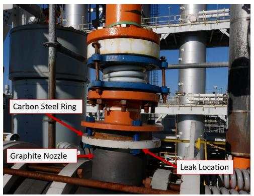
**Figure 7.** Location of Leak. Leak tests on the heat exchanger revealed a leak from the graphite nozzle underneath a carbon steel ring used to attach the nozzle to carbon steel piping. (Credit: CSB)
