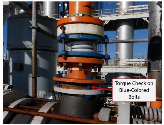
**Figure 4.** Torque check location. A Jake Marshall employee was checking the blue bolts in the image when the release occurred. (Credit: CSB)
