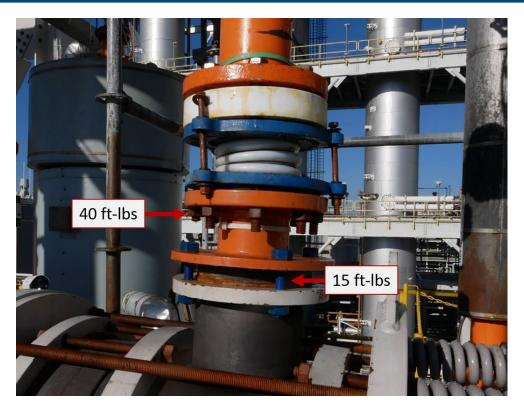
**Figure 8.** Bolt torque requirements. Two sets of bolts on the vapor outlet nozzle of the heat exchanger have different torque requirements. (Credit: CSB)
