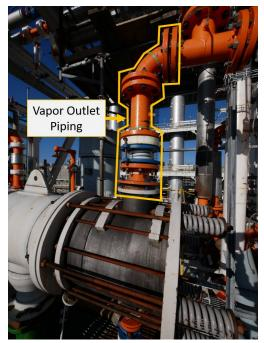
**Figure 2.** Jake Marshall Scope of Work. Wacker employees verbally requested the Jake Marshall employees check the torque on all of the bolts on the heat exchanger vapor outlet piping, which had been installed earlier in the week. (Credit: CSB)
