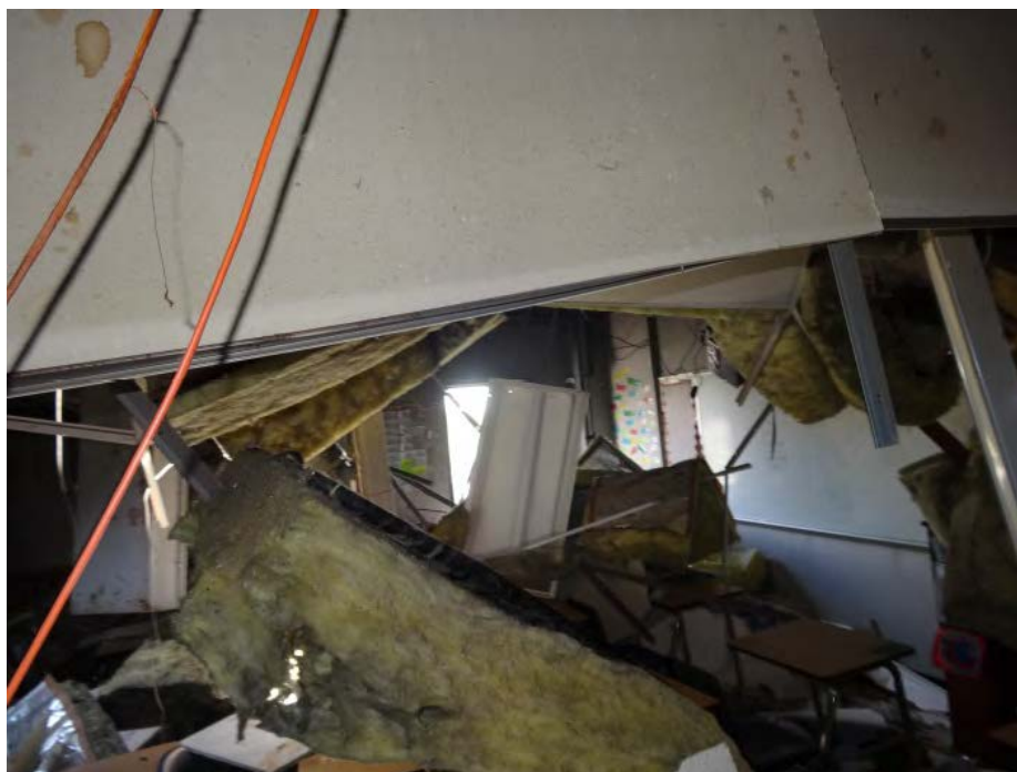
Figure 25. Glazing Hazard in WIS Room 12 (Source: ABS Consulting)
