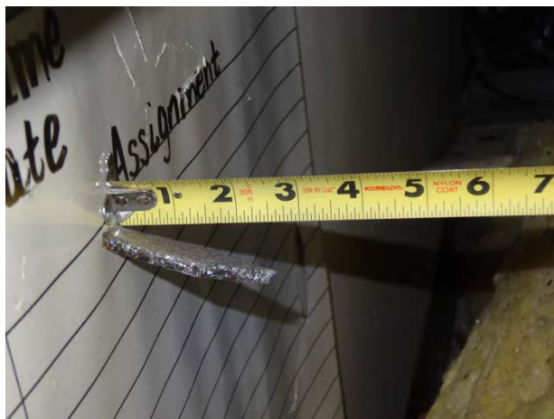
Figure 26. Embedded Glass in Assignment Poster in WIS Room 12 (Source: ABS Consulting)
