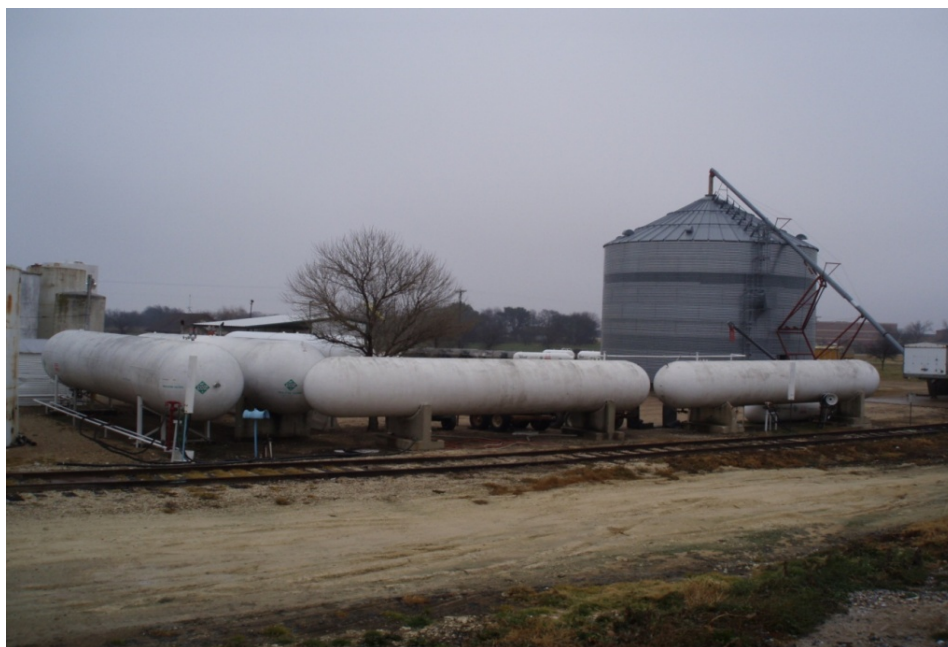
Figure 6. Anhydrous Ammonia Storage (Source: WFC Insurer)
