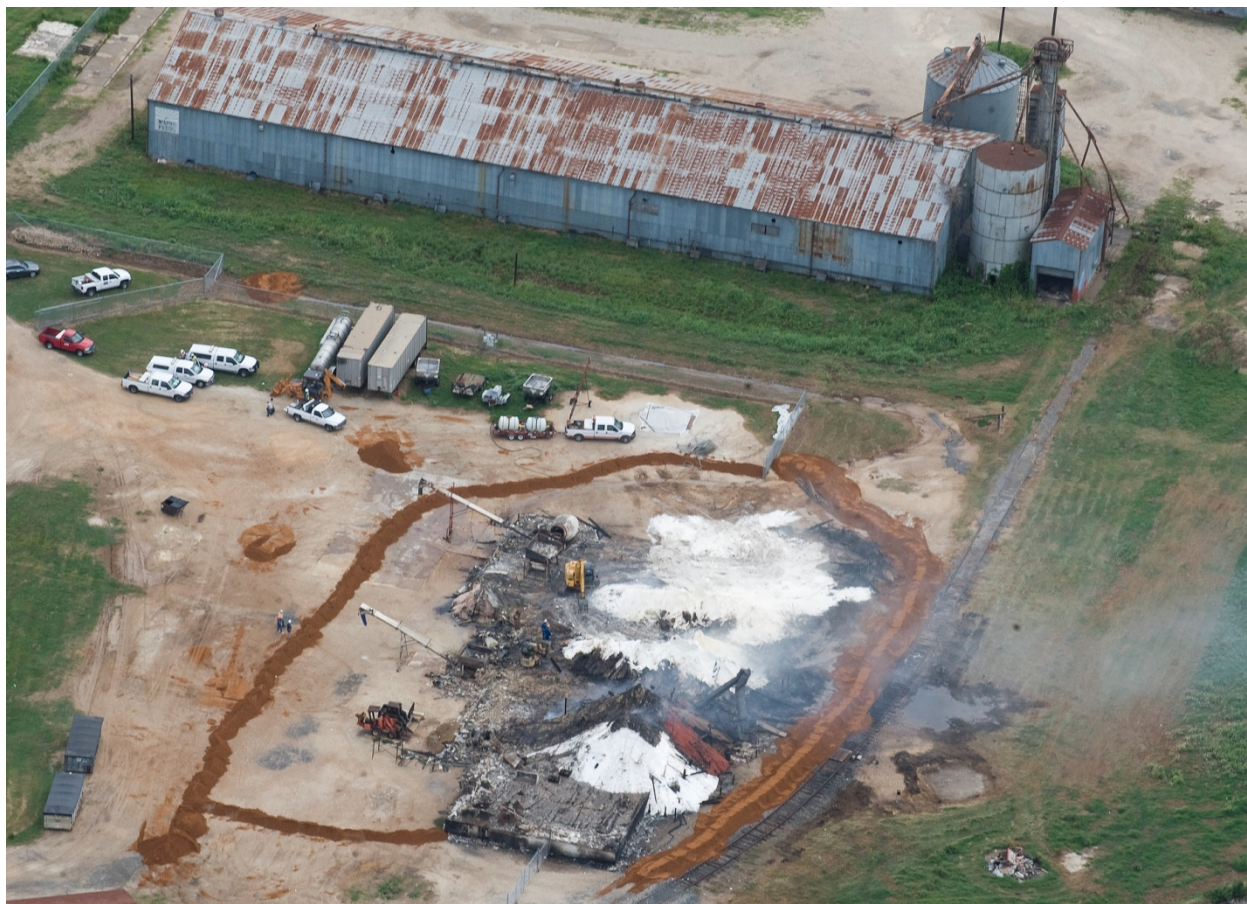
Figure 65. Post-Incident Aerial View of EDC Facility Wooden Fertilizer Warehouse (Source: Bryan-College Station Eagle)
