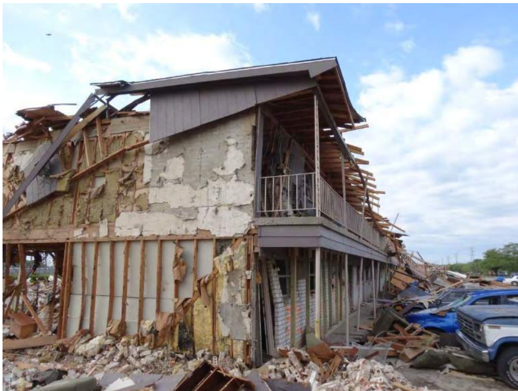
Figure 106. Apartment Complex Damage
