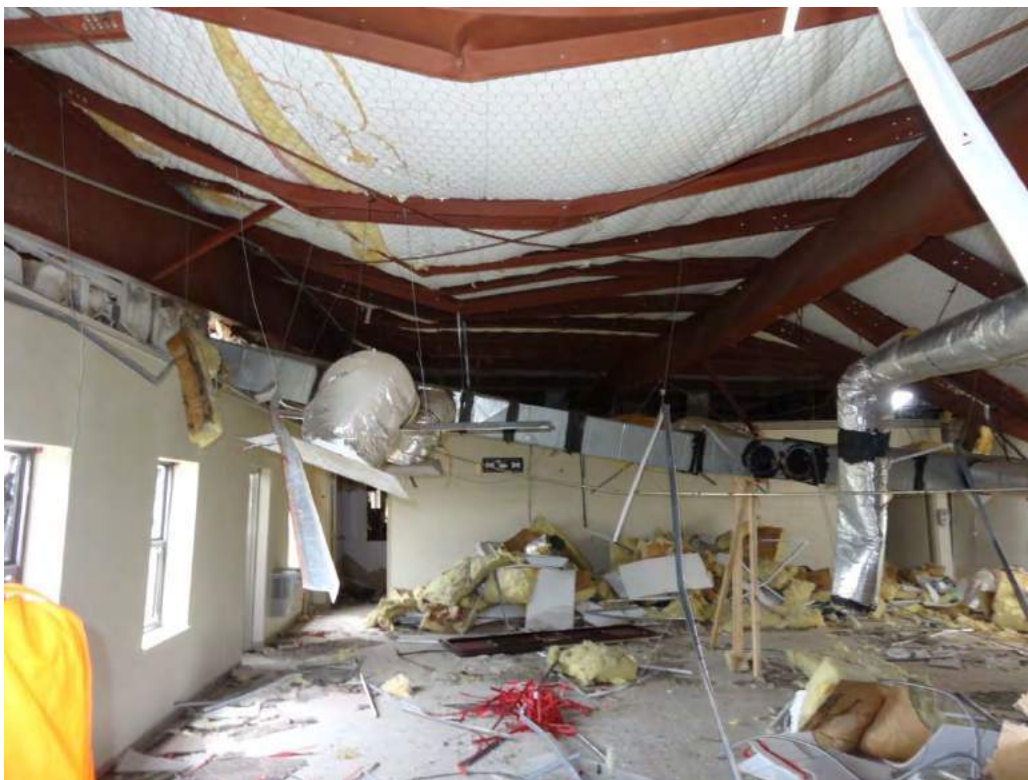
Figure 119. Roof Purlin Deformation at Gymnasium
