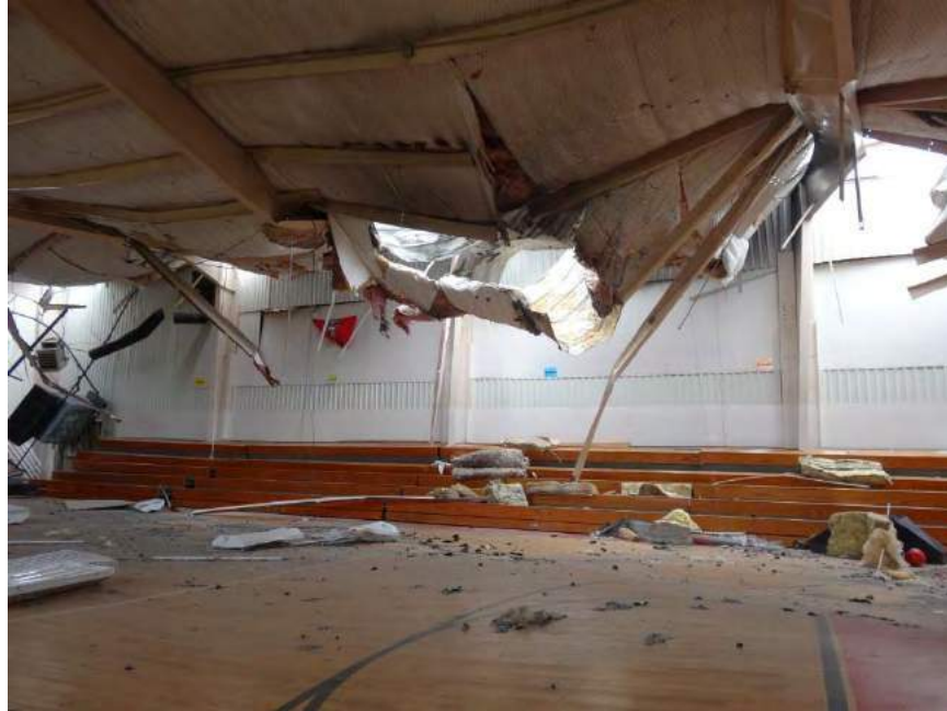
Figure 53. West Intermediate School Gymnasium Roof Failure
