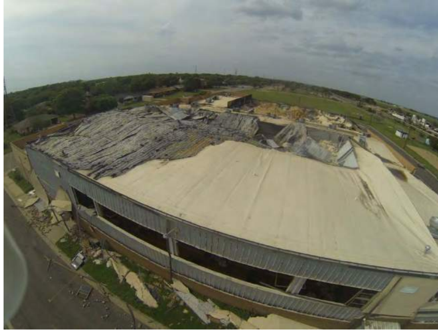
Figure 51. West Intermediate School – Gymnasium Roof
