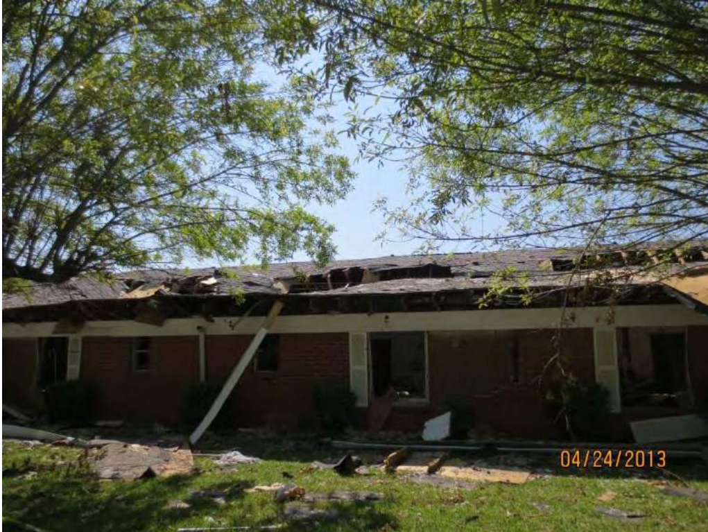
Figure 28. East Façade of North Wing Rooms at Rest Haven Nursing Home
