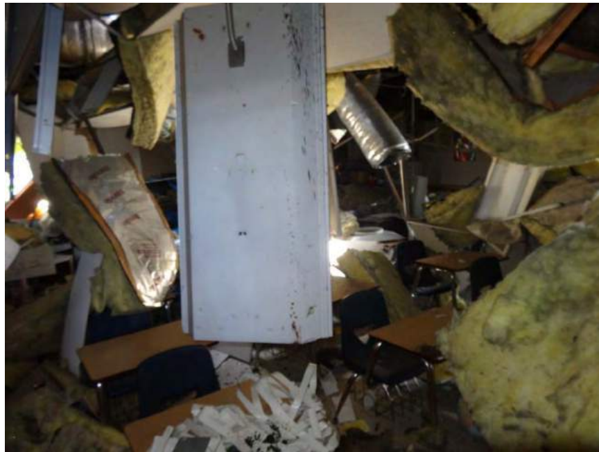
Figure 47. West Intermediate School Classroom 12
