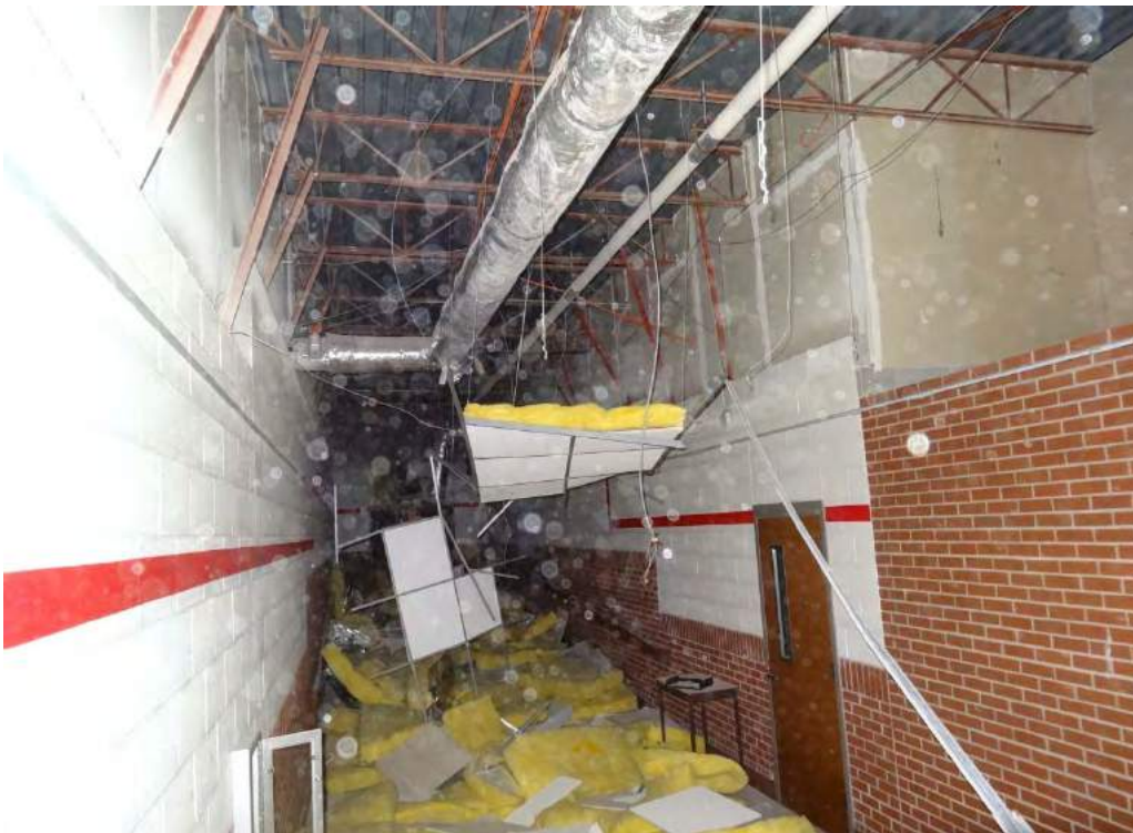
Figure 75. West High School Hallway Outside Room 411
