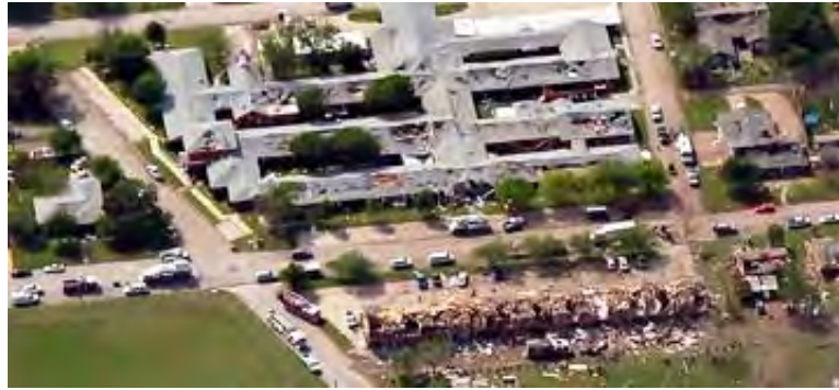
Figure 32. Post Incident Aerial View of Rest Haven Nursing Home (Debris Impacts)
