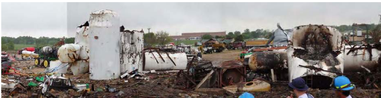
Figure 18. Liquid Fertilizer Tank Damage (Composite of three photographs)
