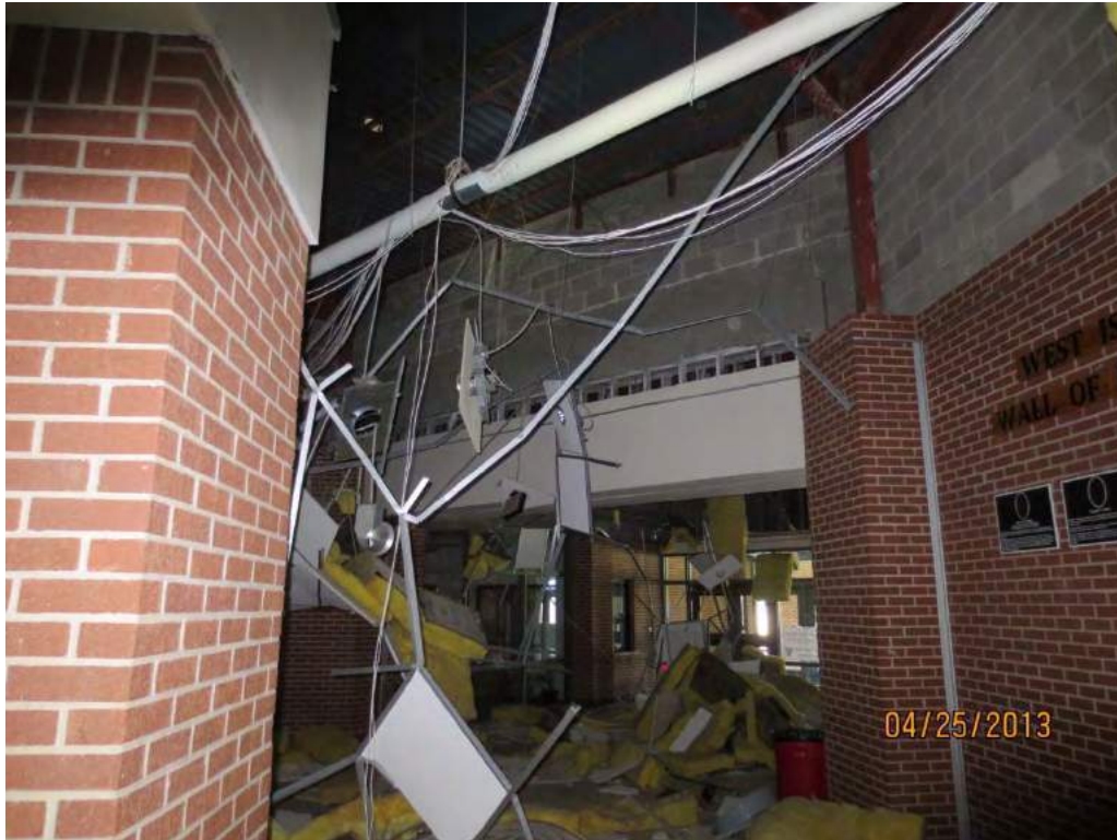
Figure 73. West High School Entrance Lobby
