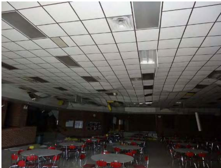
Figure 63. Commons Area Ceiling Damage
