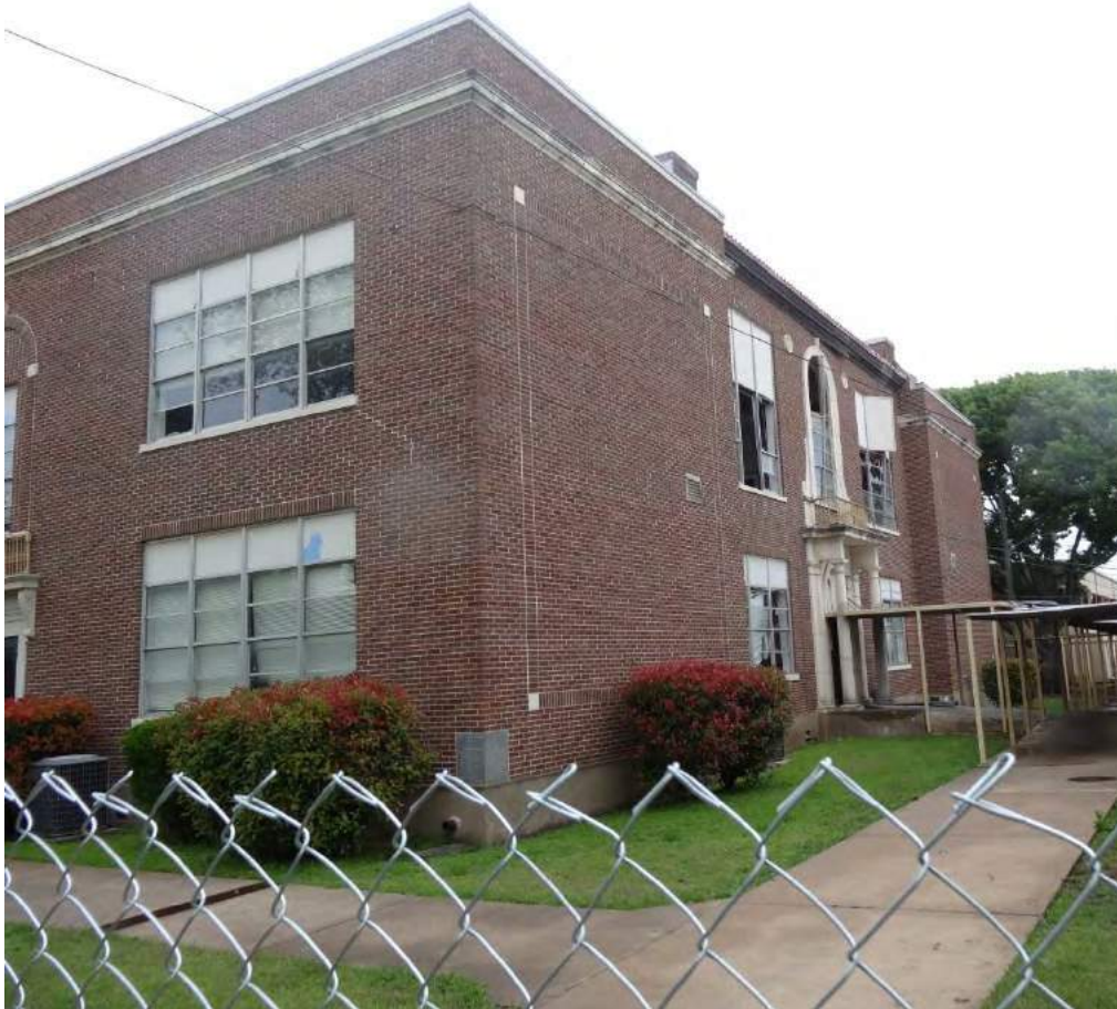
Figure 81. West Middle School – Old High School Classroom Building
