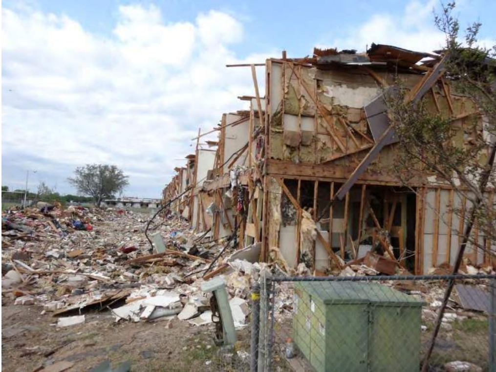
Figure 107. Apartment Complex Damage
