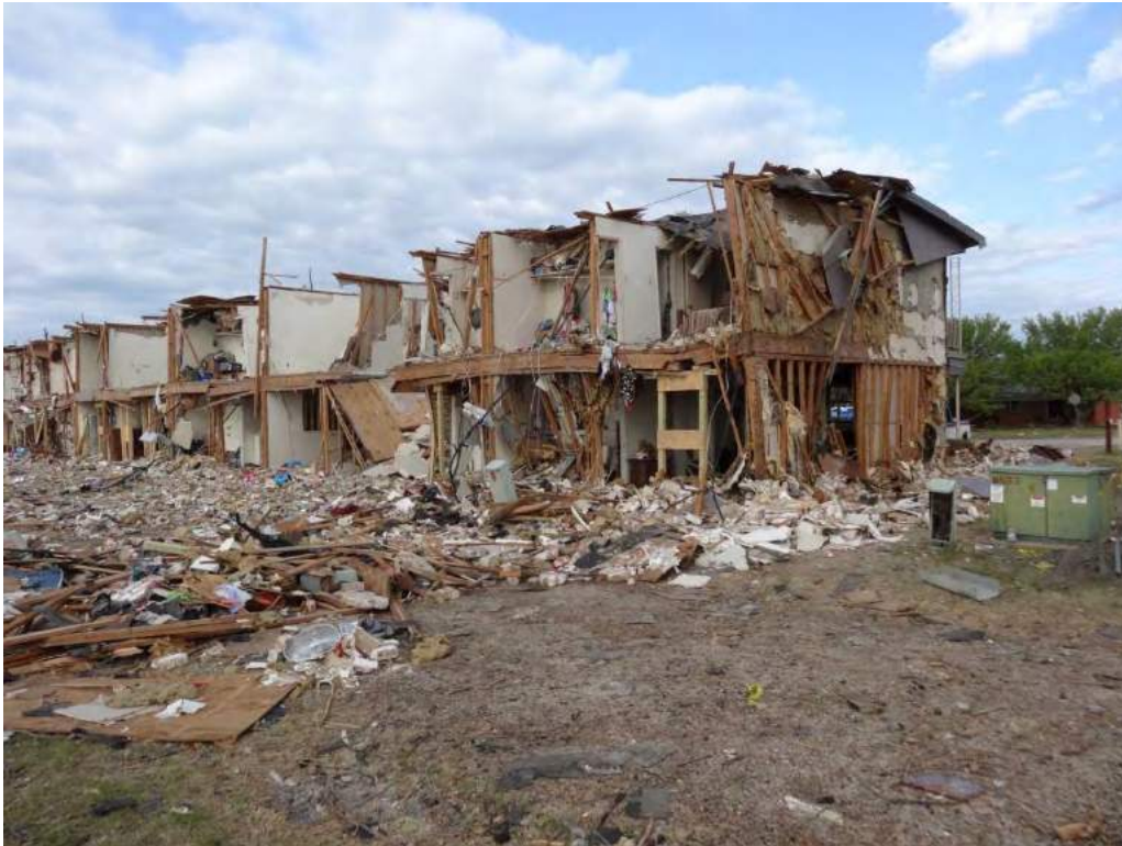
Figure 86. Apartment Complex East Façade
