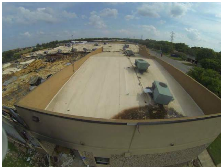
Figure 45. West Intermediate School – Northwest Wing Roof
