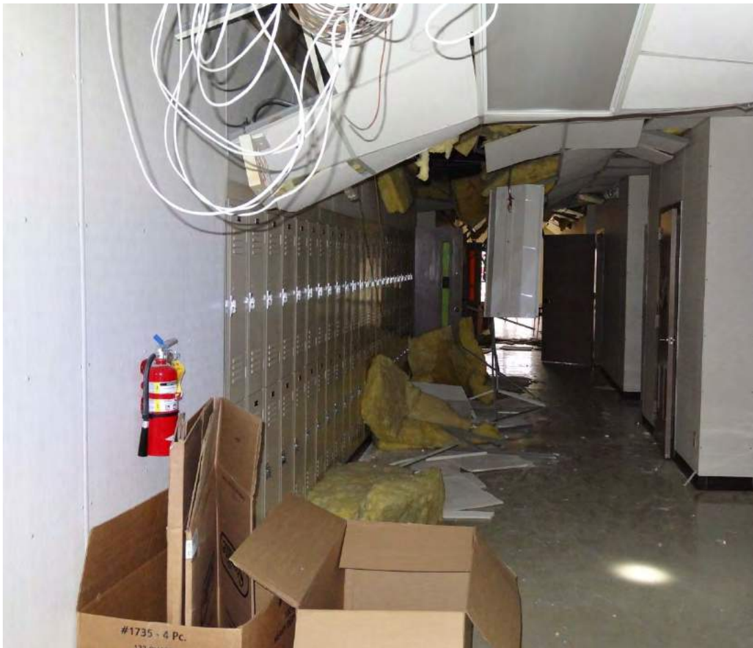
Figure 83. Classroom Annex Interior Hallway and Ceiling Damage
