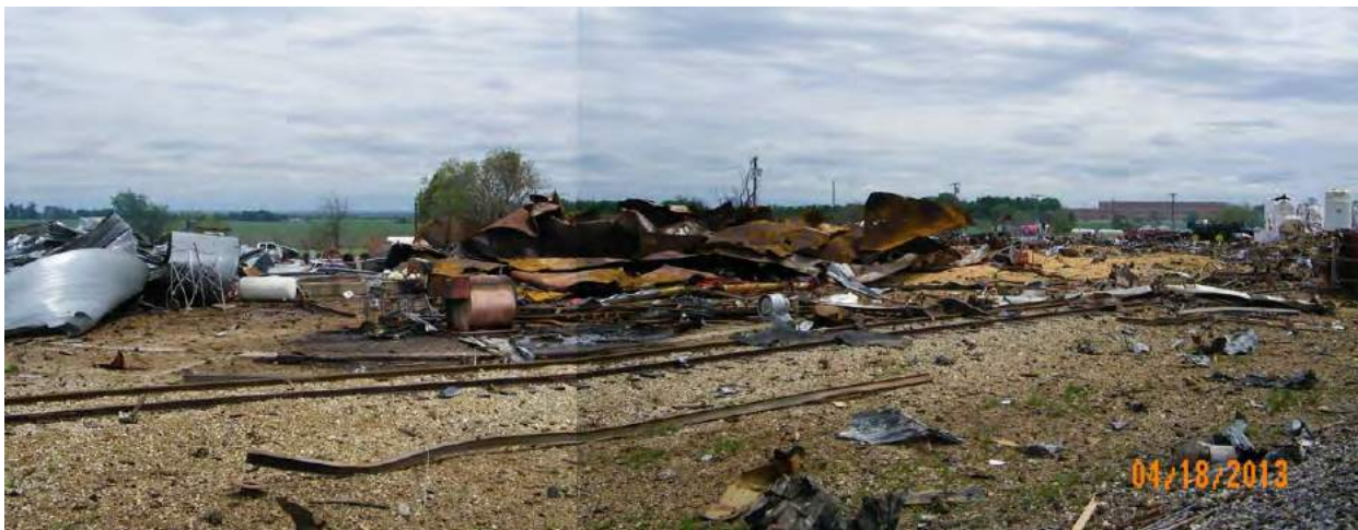
Figure 16. Corn Silo Damage (Composite of Two Photographs)
