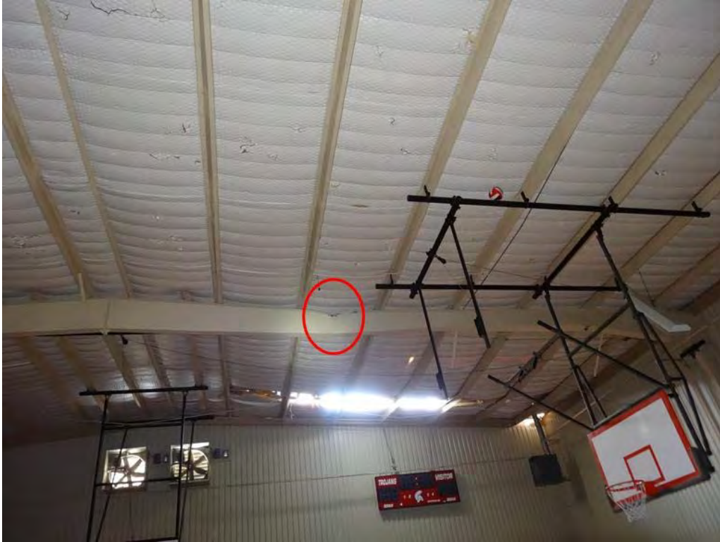
Figure 79. West Middle School Practice Gym Buckled Frame
