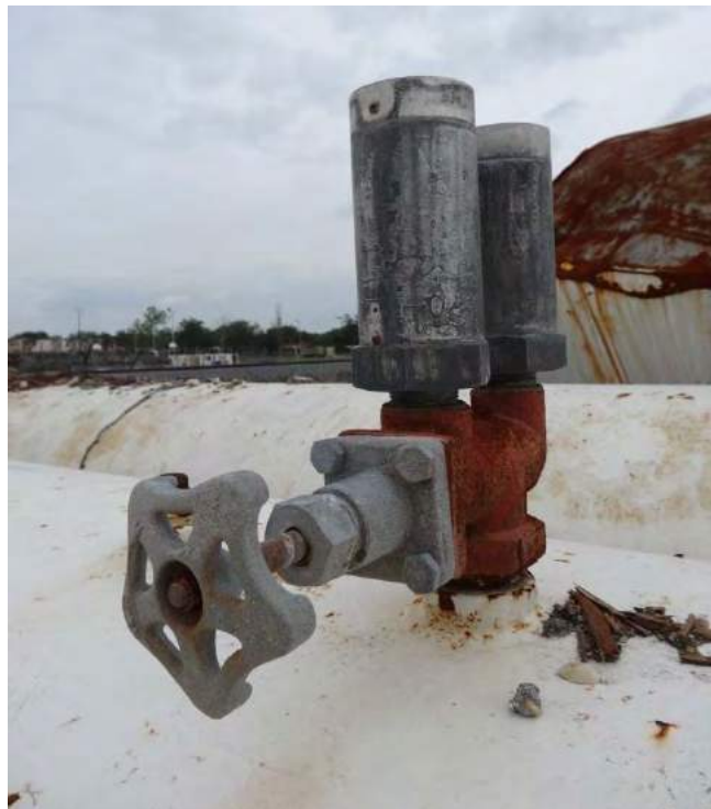
Figure 20. PRV Valve from Southern Anhydrous Ammonia Tank (Photo 05-28-13)
