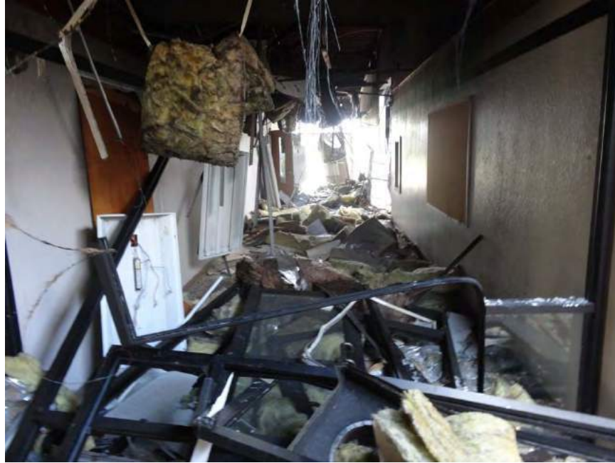
Figure 46. West Intermediate School- North Hallway Looking Toward Northeast Exit Door
