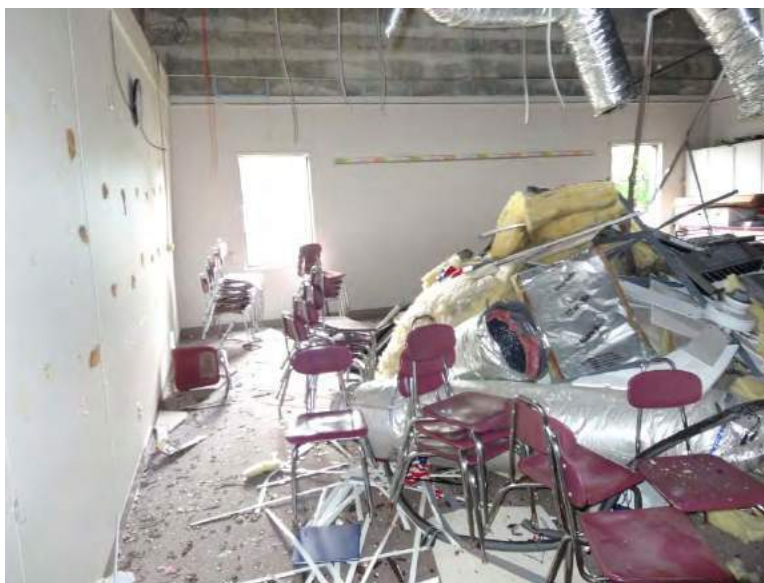
Figure 58. West Intermediate School Room 22 Interior after Moderate Cleanup
