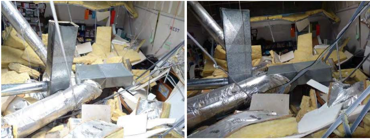
Figure 55. West Intermediate School – Classroom 20 Nonstructural Debris
