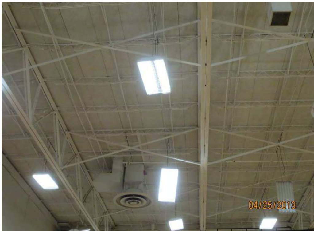
Figure 67. Buckled OWSJs in Gymnasium 2
