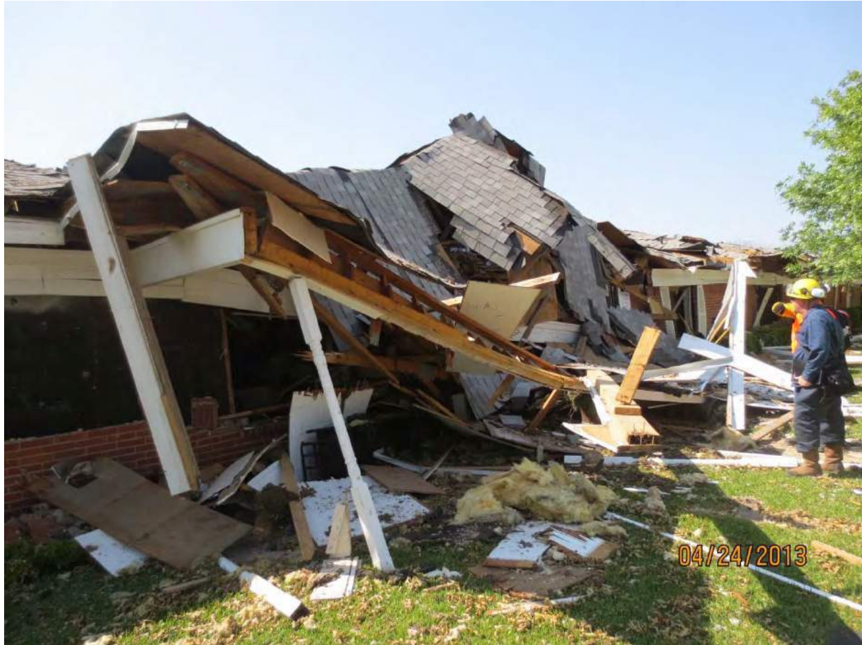
Figure 27. Damage to Reagan St. Entry of Rest Haven Nursing Home
