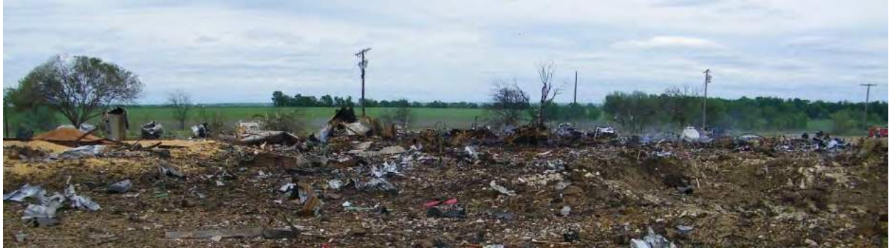
Figure 15. Remains of Chemical Storage / Office Building (Behind Crater in Photo)
