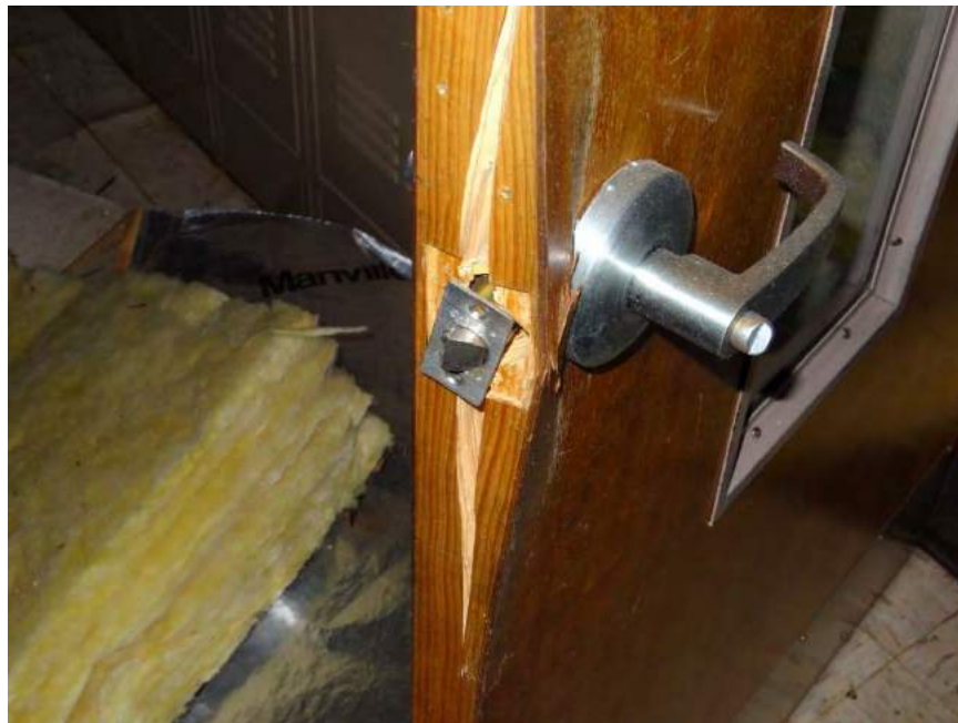
Figure 56. West Intermediate School – Typical Failed Classroom Door Latch
