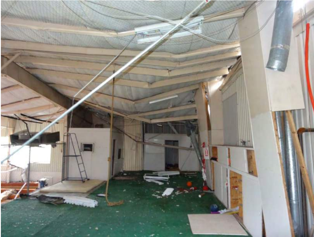
Figure 119. Roof Purlin Deformation at Gymnasium
