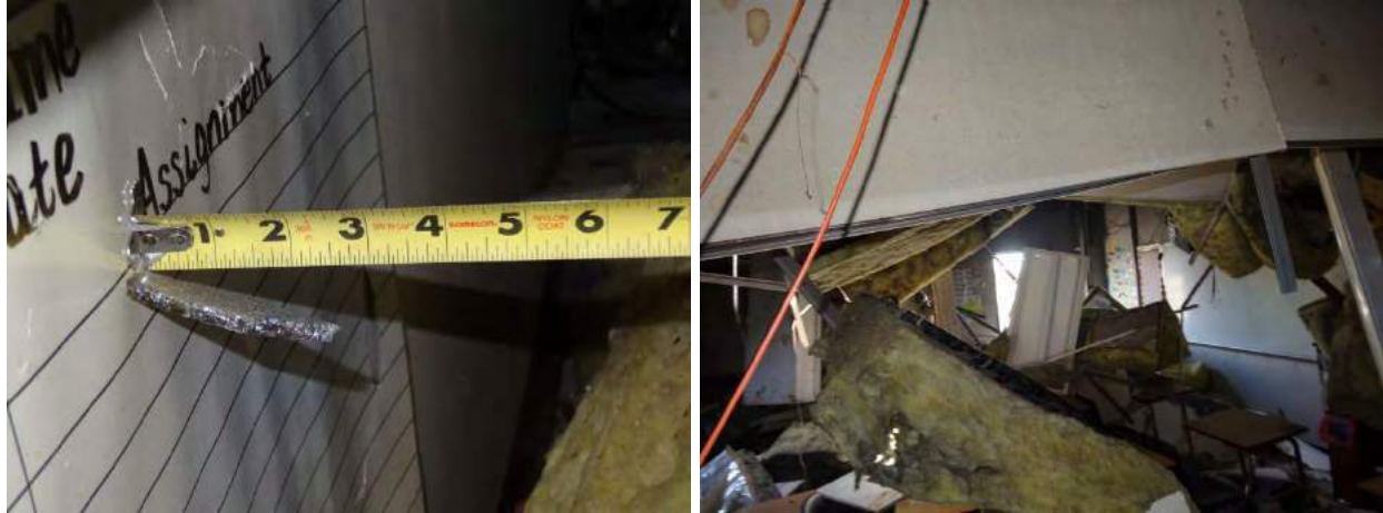
Figure 48. West Intermediate School Glazing Hazard Room 12
