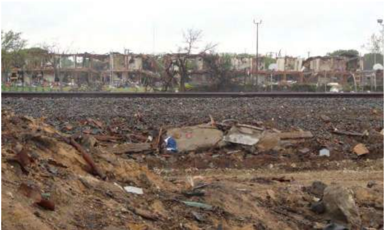
Figure 105. Apartment Complex Damage
