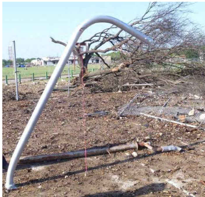
Figure 38. Damaged Basketball Goal Post on Basketball Court
