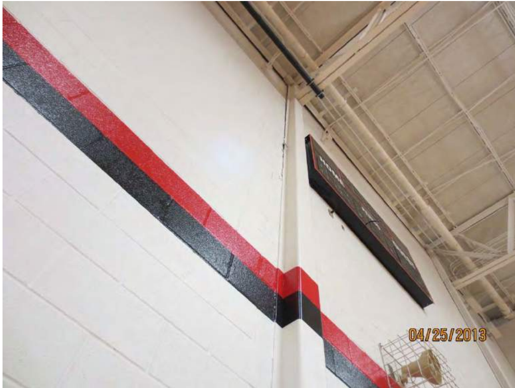
Figure 68. West Wall of Gymnasium 2
