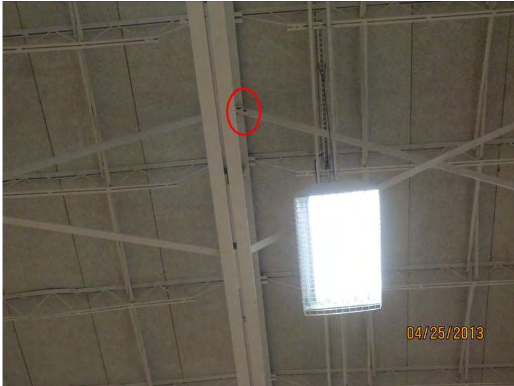
Figure 66. Failed Cross-Bracing Fasteners Gymnasium 2
