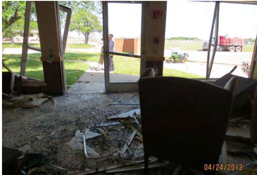
Figure 34. Typical Glass Fragments on Floor and Into Rooms of Rest haven Nursing Home
