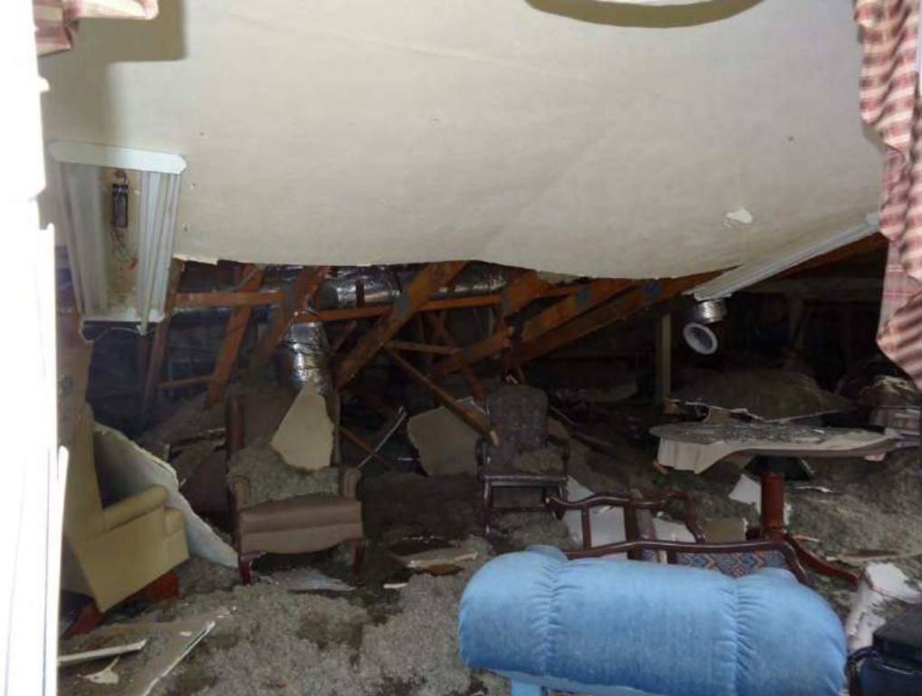
Figure 30. West Lobby of Rest Haven Nursing Home
