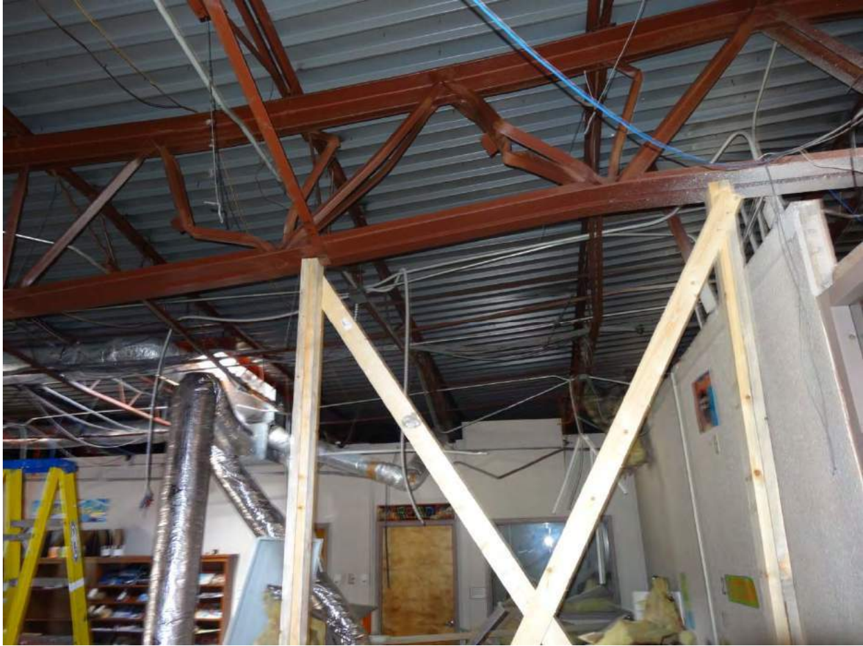
Figure 122. Joist Girder Deformation at Library
