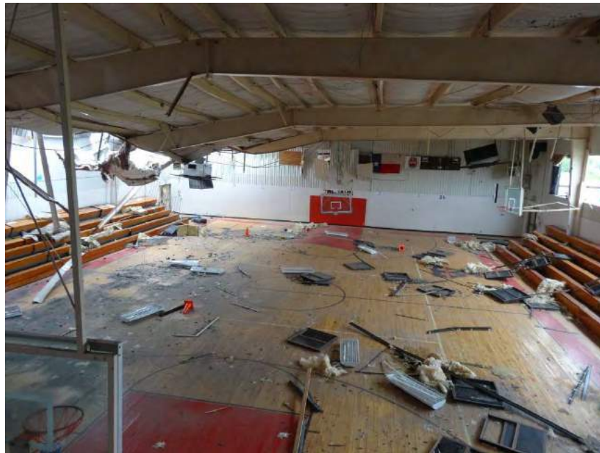
Figure 52. West Intermediate School Gymnasium
