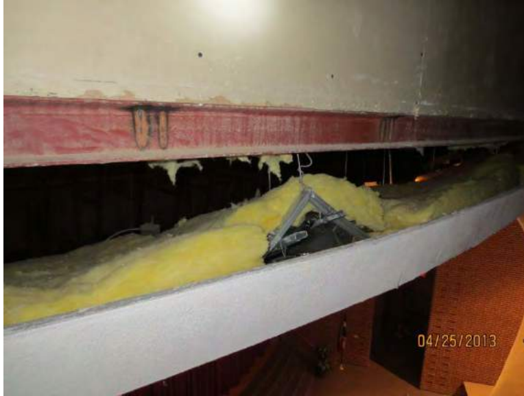
Figure 62. Auditorium Ceiling Hanger Damage
