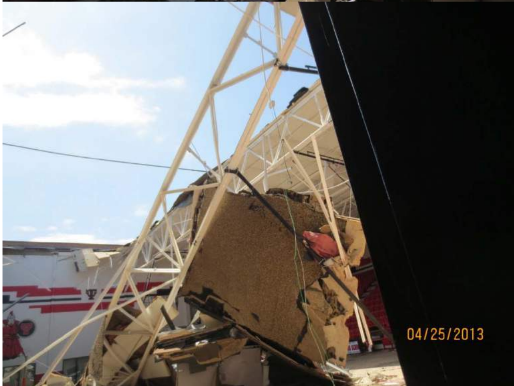
Figure 71. West high School Gymnasium1 Roof Collapse Viewed from Gymnasium Floor Entry
