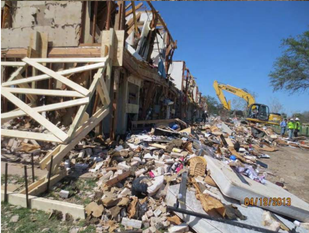
Figure 87. Apartment Complex after USAR Operations
