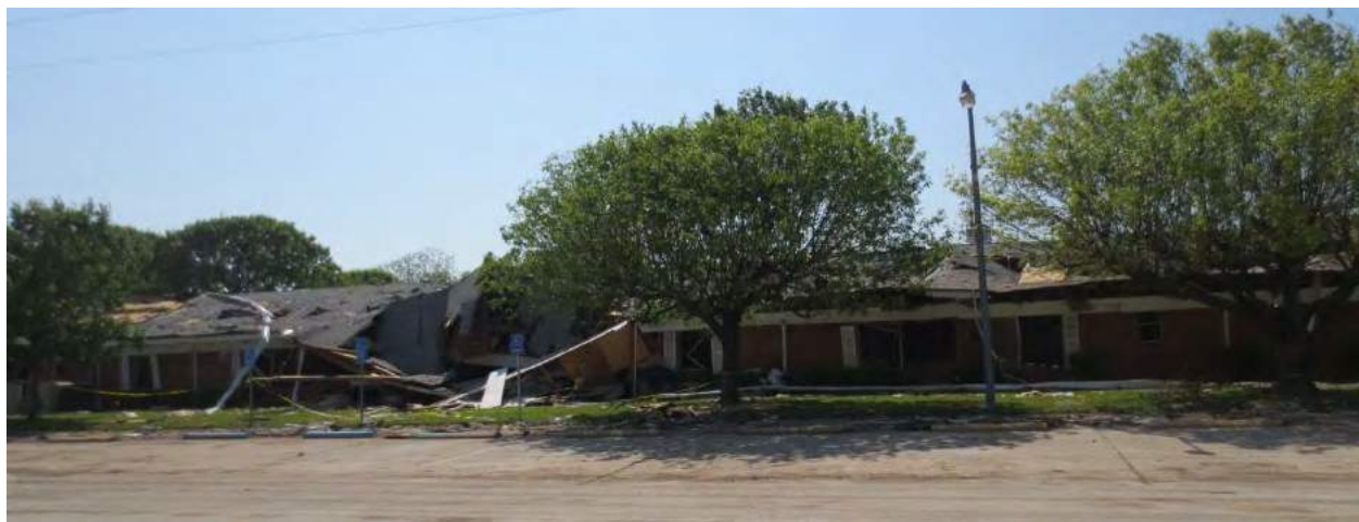
Figure 26. East Façade of Rest Haven Nursing Home
