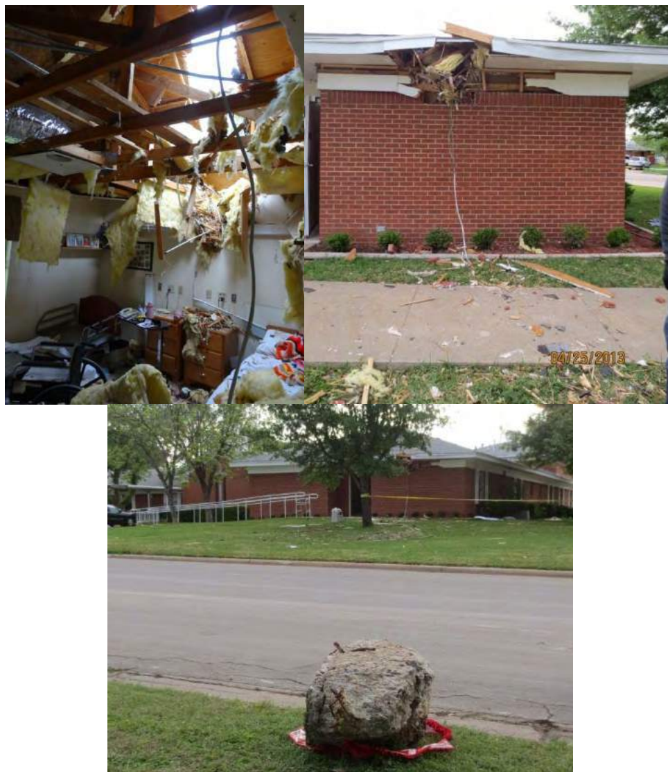
Figure 33. Concrete Crater Debris (West Fertilizer Foundation) that Impacted Nursing Home
