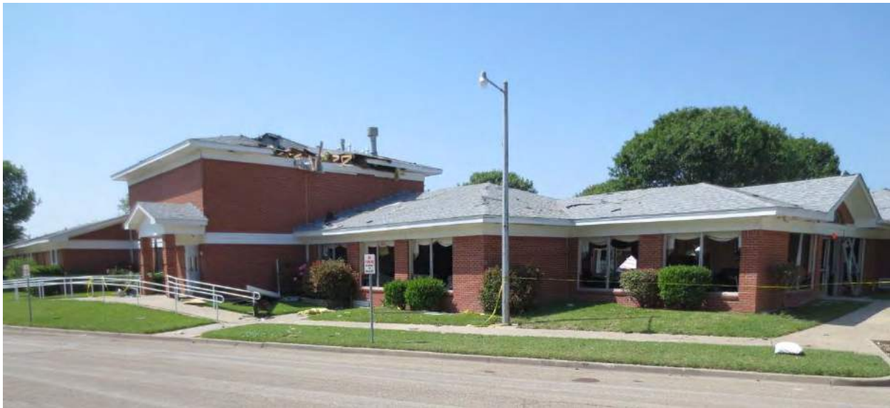
Figure 24. Rest Haven Nursing Home
