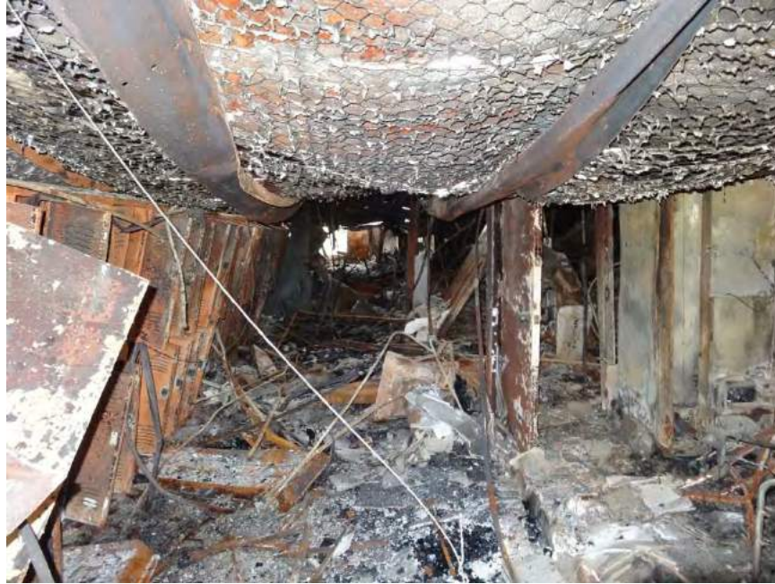
Figure 50. West Intermediate School Interior of Northeast Section that Burned
