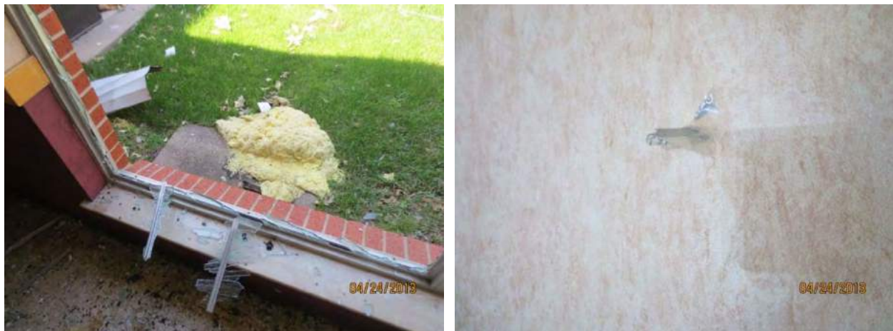
Figure 35. Typical High Glazing Hazards in Rest Haven Nursing Home
