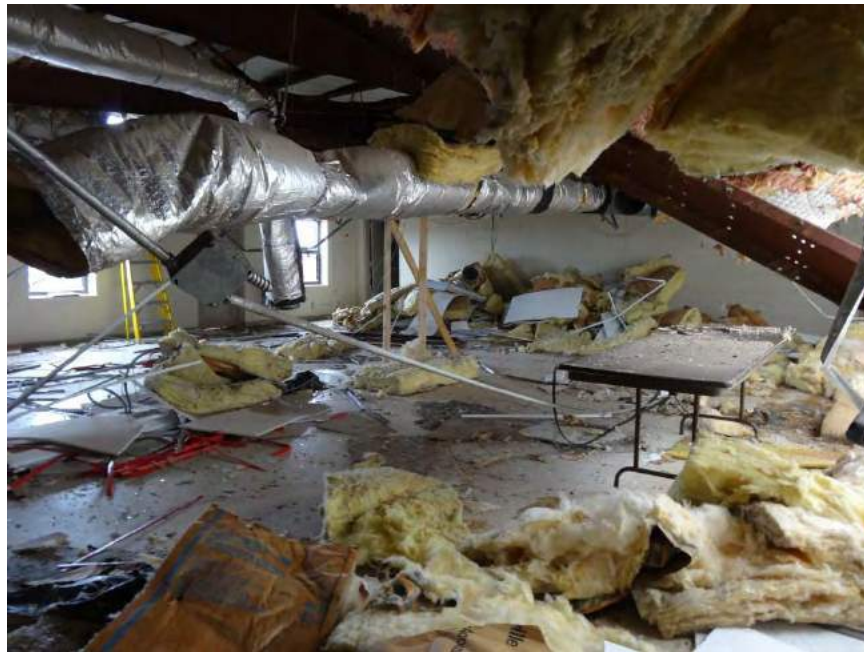
Figure 54. West Intermediate School Cafeteria (Insulate has been picked up and stacked)
