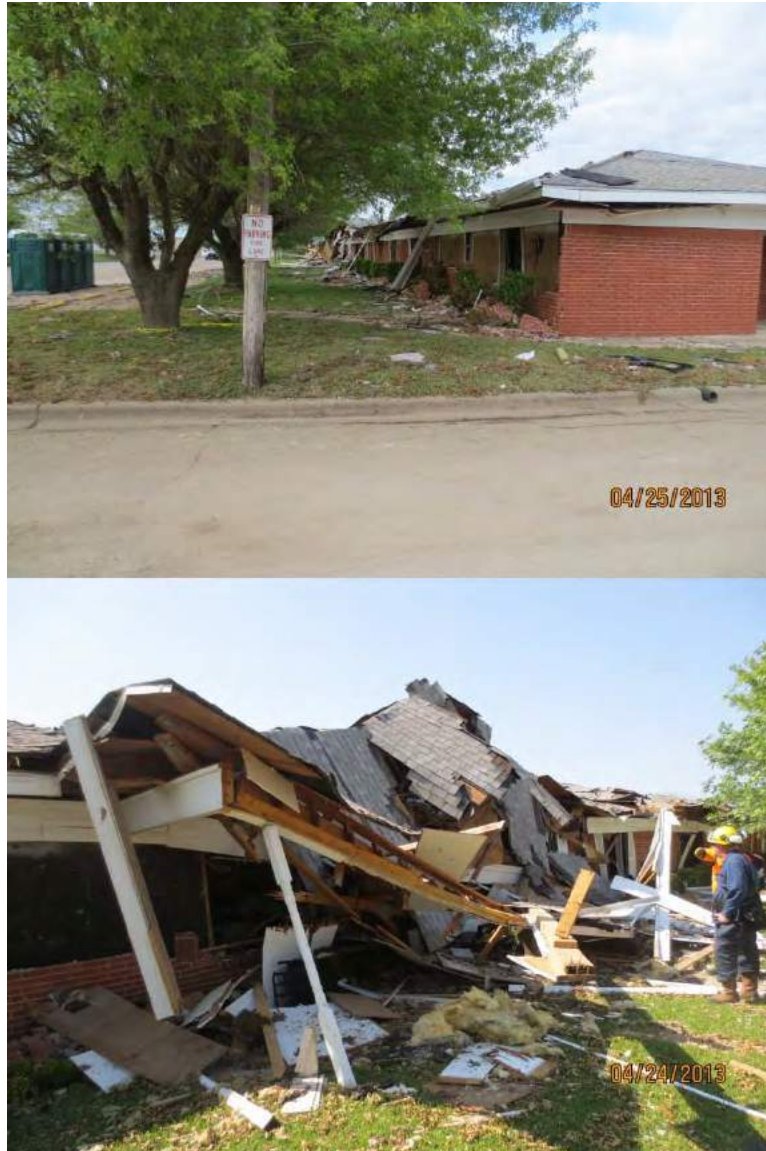
Figure 109. Rest Haven Nursing Home East Façade Damage
