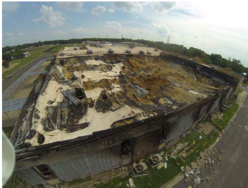
Figure 49. West Intermediate School – Original School Northeast Wing Roof
