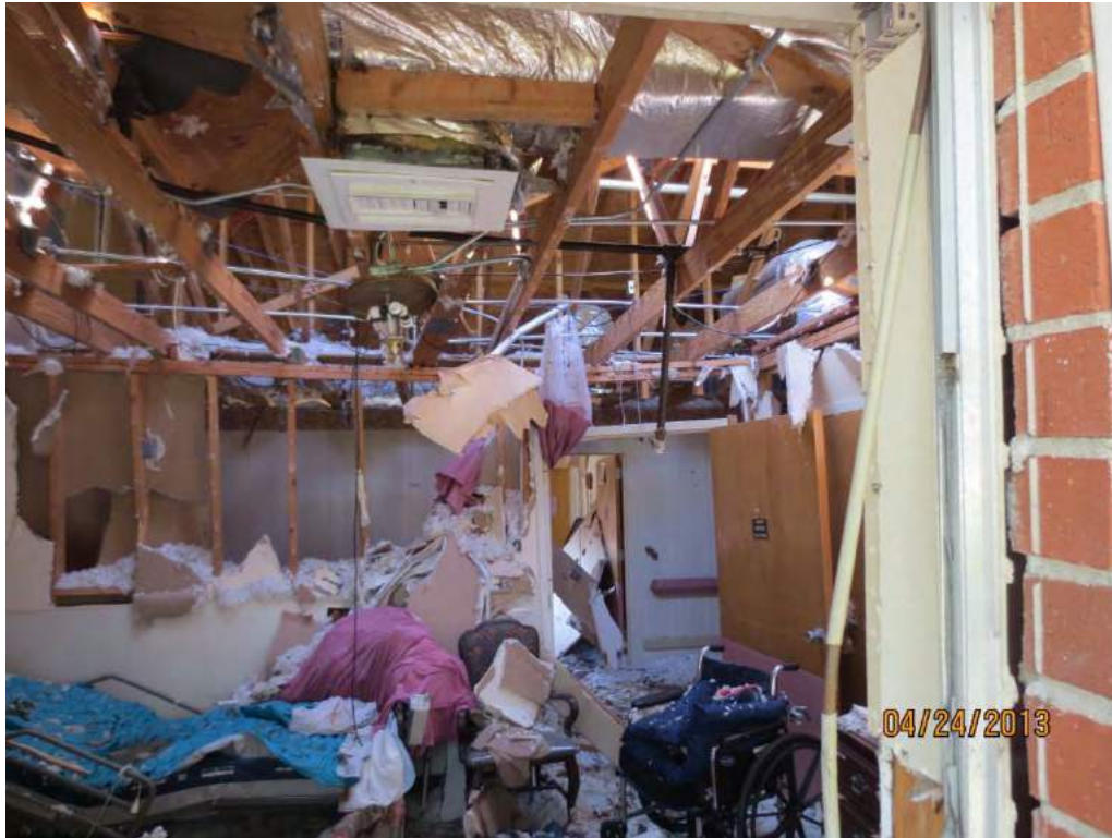
Figure 29. East Façade Bedroom in Rest Haven Nursing Home (After FEMA USAR Operations)
