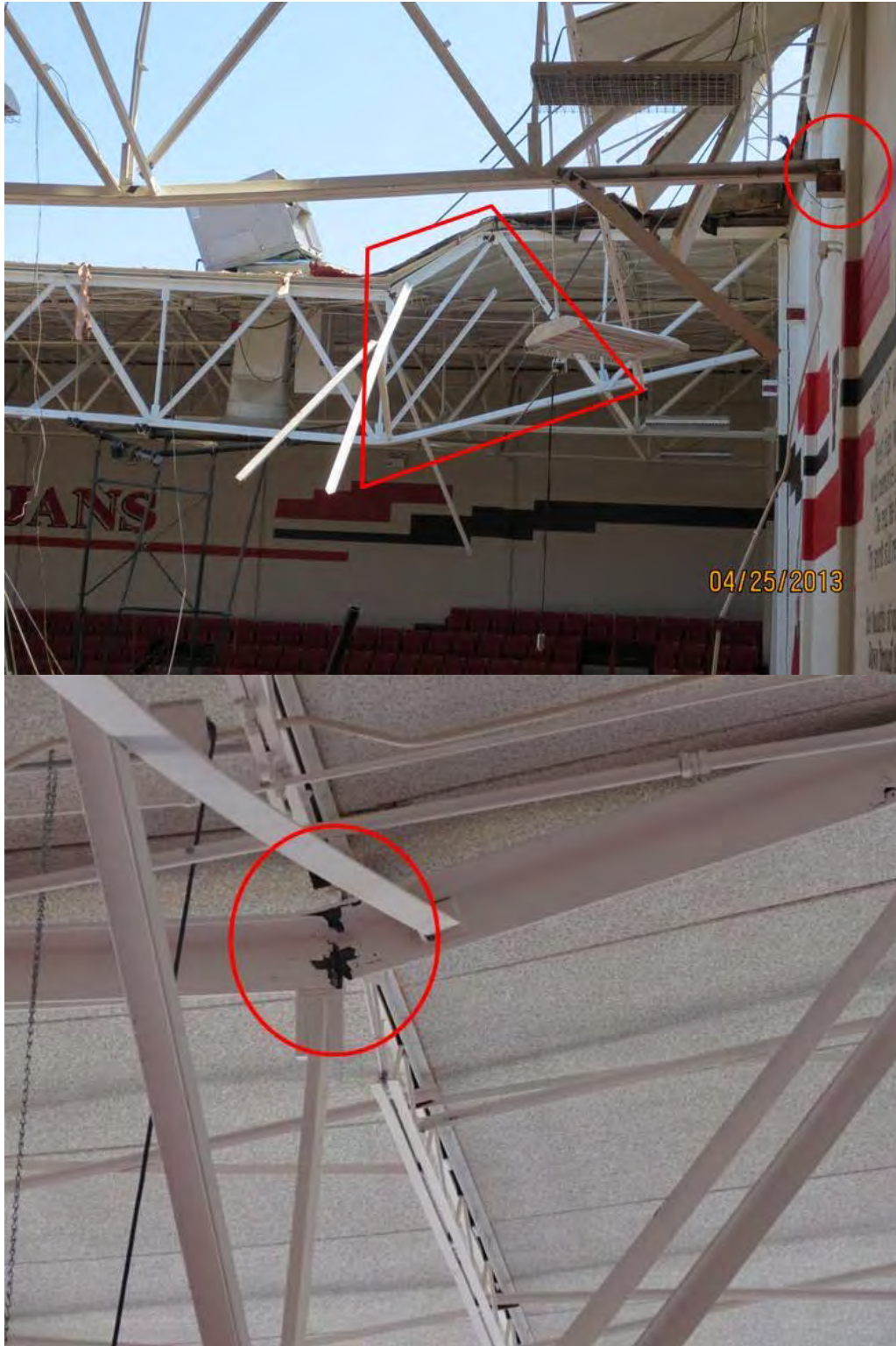
Figure 72. Joist Girder Damage in Gymnasium 1
