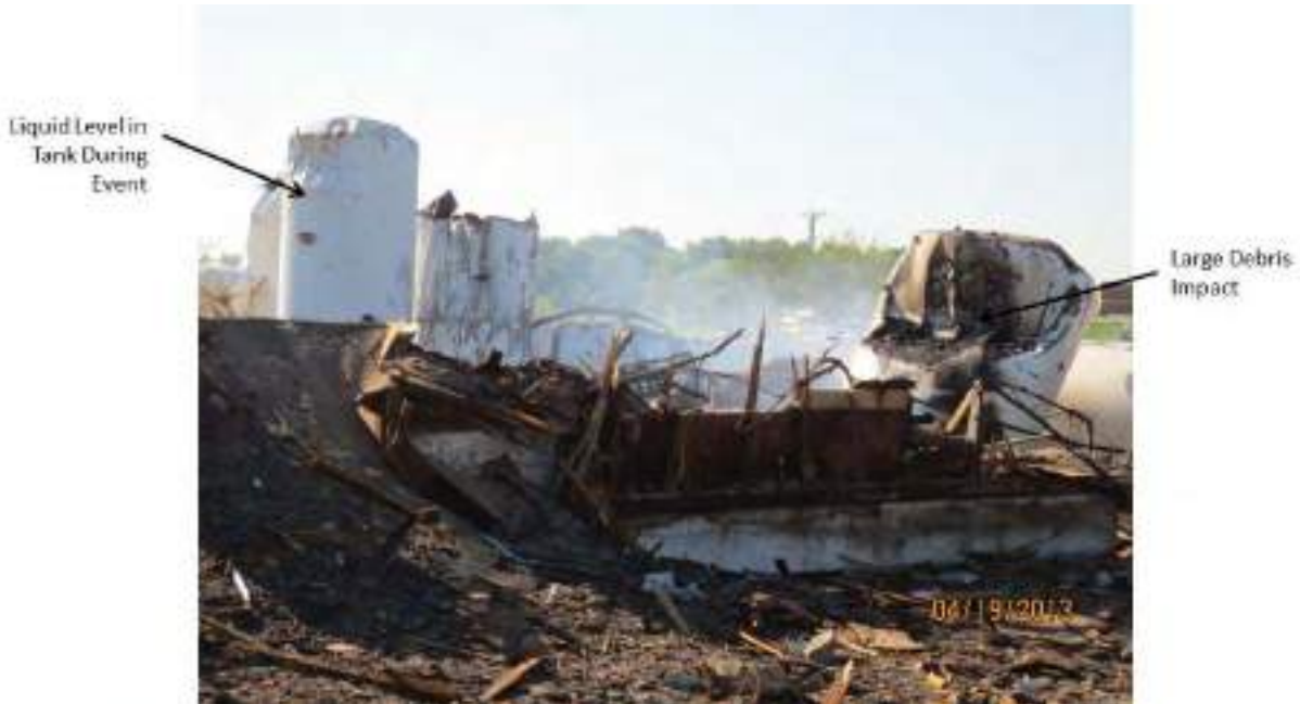
Figure 17. Liquid Fertilizer Tank Damage
