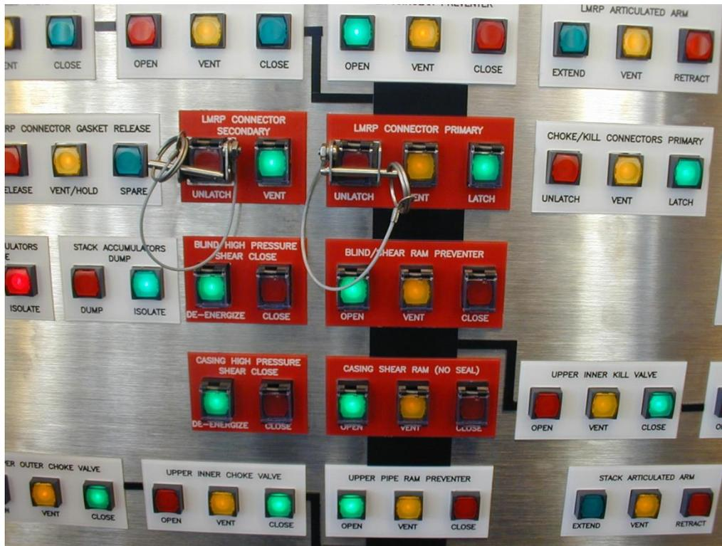
Figure 3. Portion of the control pushbutton panel for the BOP.<sup>28</sup>
