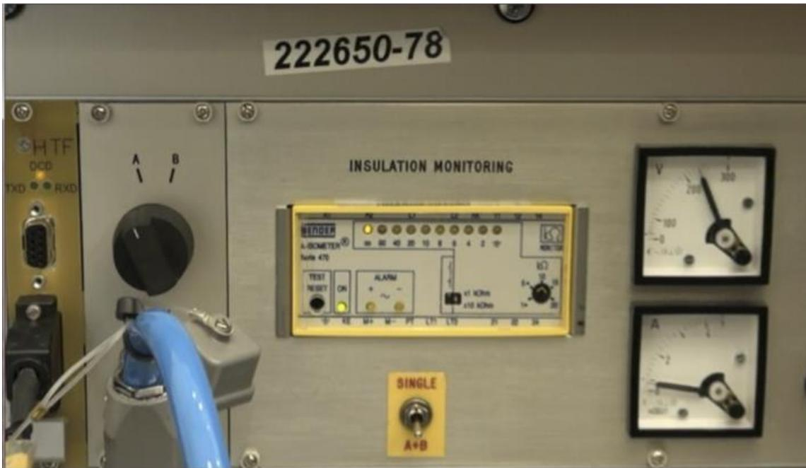
Figure 8. PETU: Note the A/B switch and the Single/A+B switch - Photo Phase 2 testing
