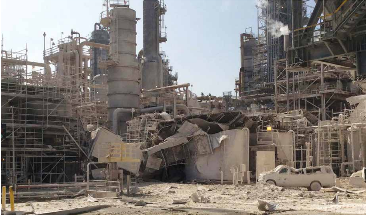
A view of the Exxon Refinery in Torrance, CA, following a 2015 explosion.
