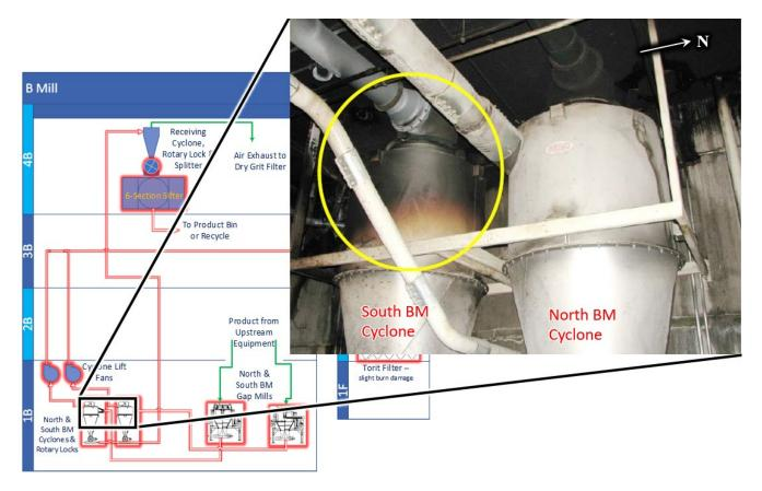
**Figure 29:** Some of North (right) and South (left) BM Cyclones' burn damage in 1B, circled. (Credit: Didion inset; CSB background and annotations)
