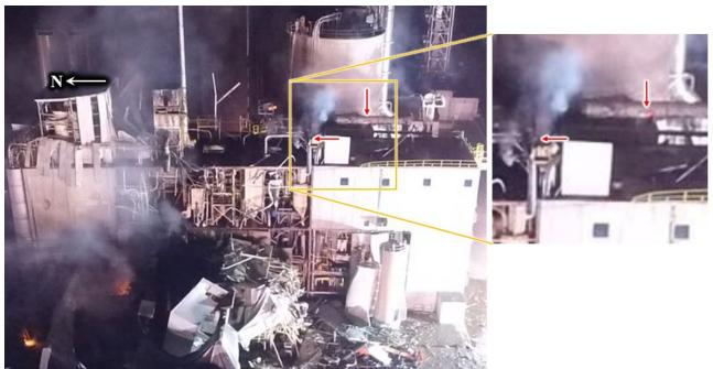
**Figure 51:** Dry Grit Filter ductwork on fire (red arrows) hours after the explosions. Inset: close-up of ductwork. (Credit: Columbia County Sherriff's Department, annotations by CSB)
