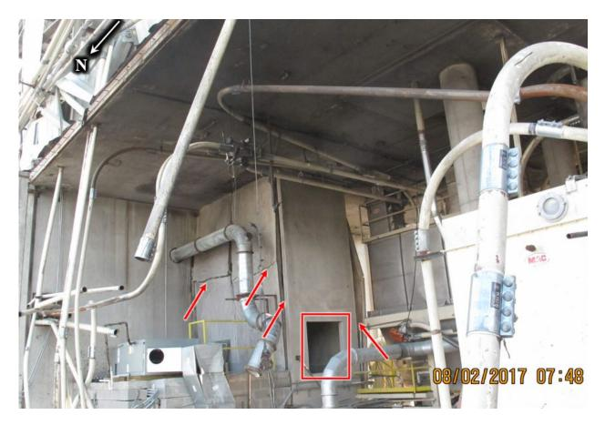
**Figure 40:** 4B air shaft damage (red arrows) and shaft opening into 4B (red box) in B Mill interior, predemolition. The 4B wall panels detached from the B Mill structure during the incident. (Credit: Didion, annotations by CSB)
