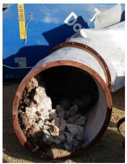
Figure 49: Torit Filter supply ducting with material deposits inside. (Credit: CSB)
