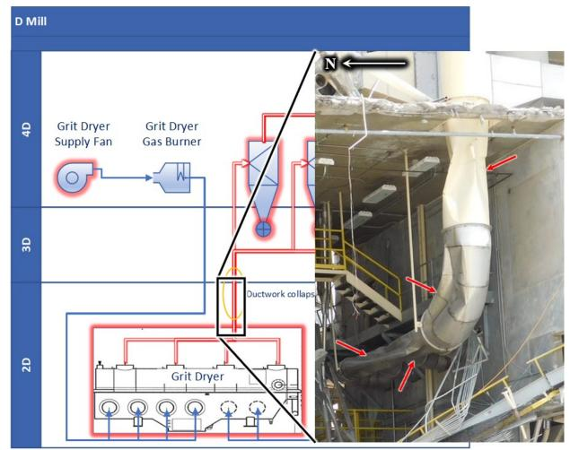
**Figure 38:** Grit Dryer exhaust ductwork in D Mill, between Grit Dryer and 4D cyclones, found collapsed post-incident (red arrows). (Credit: Didion, annotations by CSB)
