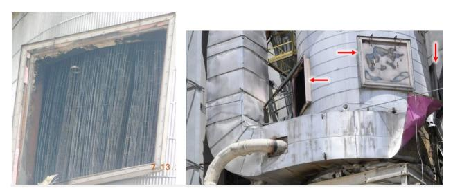
**Figure 31:** Dry Grit Filter damage. Internal damage (left). The filter socks were burned away, leaving only the metal cages. Deflagration vents (right, red arrows) stuck open and with burn damage. (Credit: Didion, annotations by CSB)
