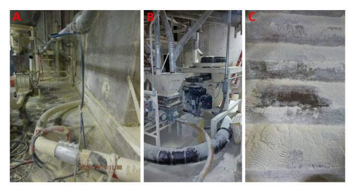
**Figure 58:** Examples of fugitive dust accumulations, (A) approximately three months before the incident, (B) approximately two weeks before the incident, and (C) less than 24 hours before the incident. (Credit: Didion)
