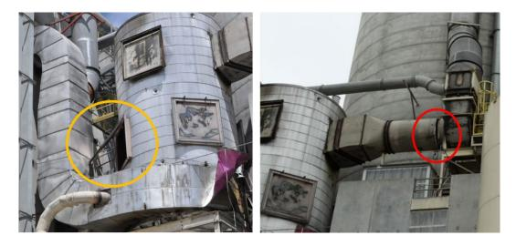
**Figure 53:** Dry Grit Filter installation. Open vent panel is denoted by the orange circle, and the exhaust ducting damage is highlighted by the red circle. (Credit: CSB)
