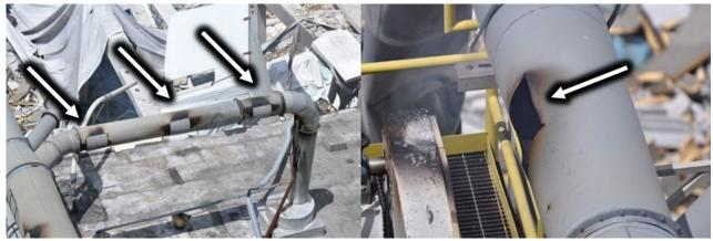
Figure 56: Dry Grit Filter ducting with overpressure indications. (Credit: CSB)
