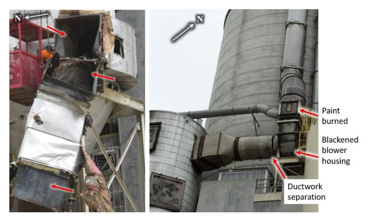
**Figure 32:** Examples of Dry Grit Filter ductwork and blower damage (red arrows). Inlet duct blackened (shown during demolition, left) and exhaust to atmosphere, including blower (right). (Credit: left, Didion with annotations by CSB; right, CSB)
