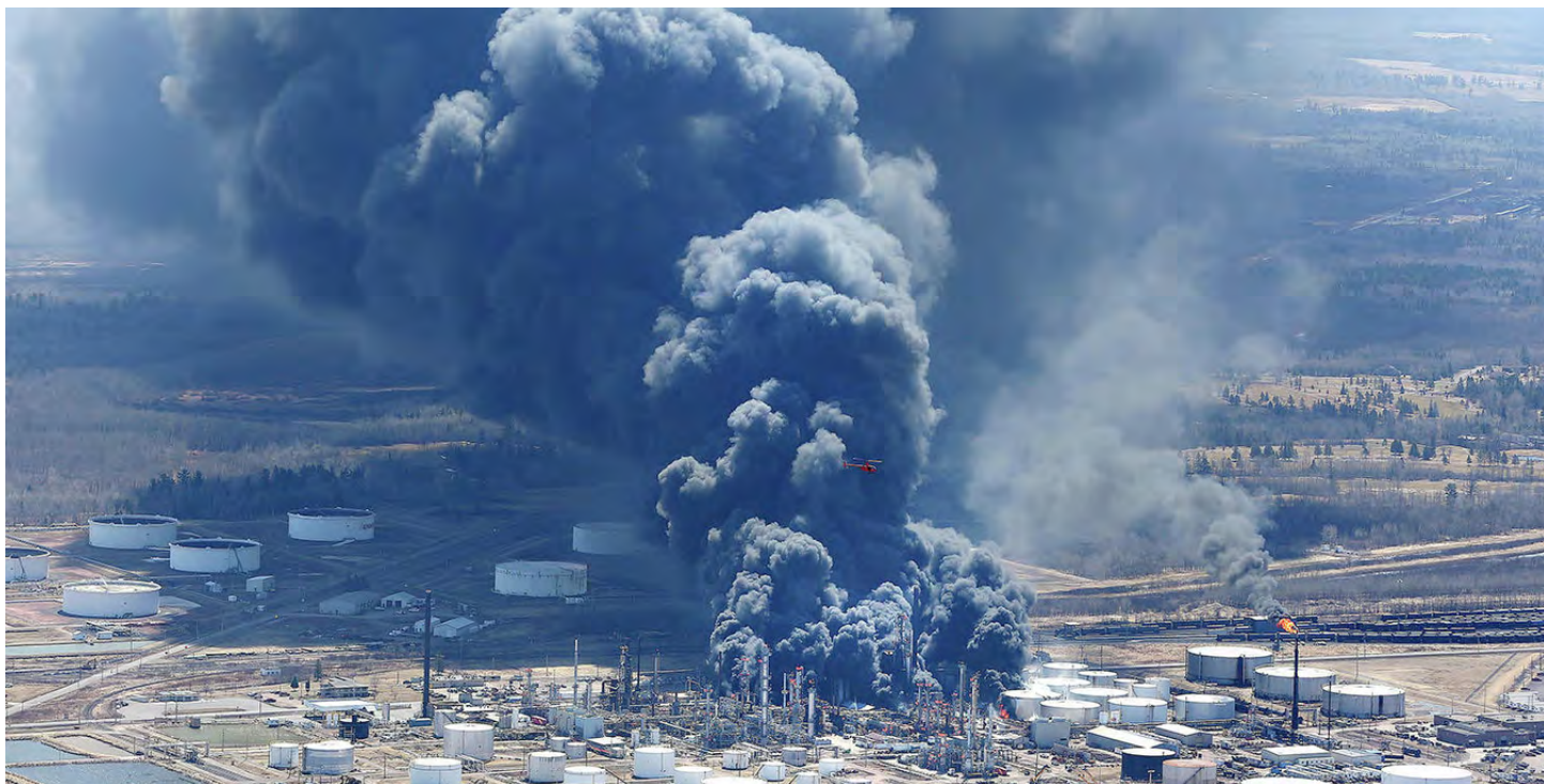
Figure 2. Smoke from the Fire at the Husky Superior Refinery. Credit: WDIO ABC News.
