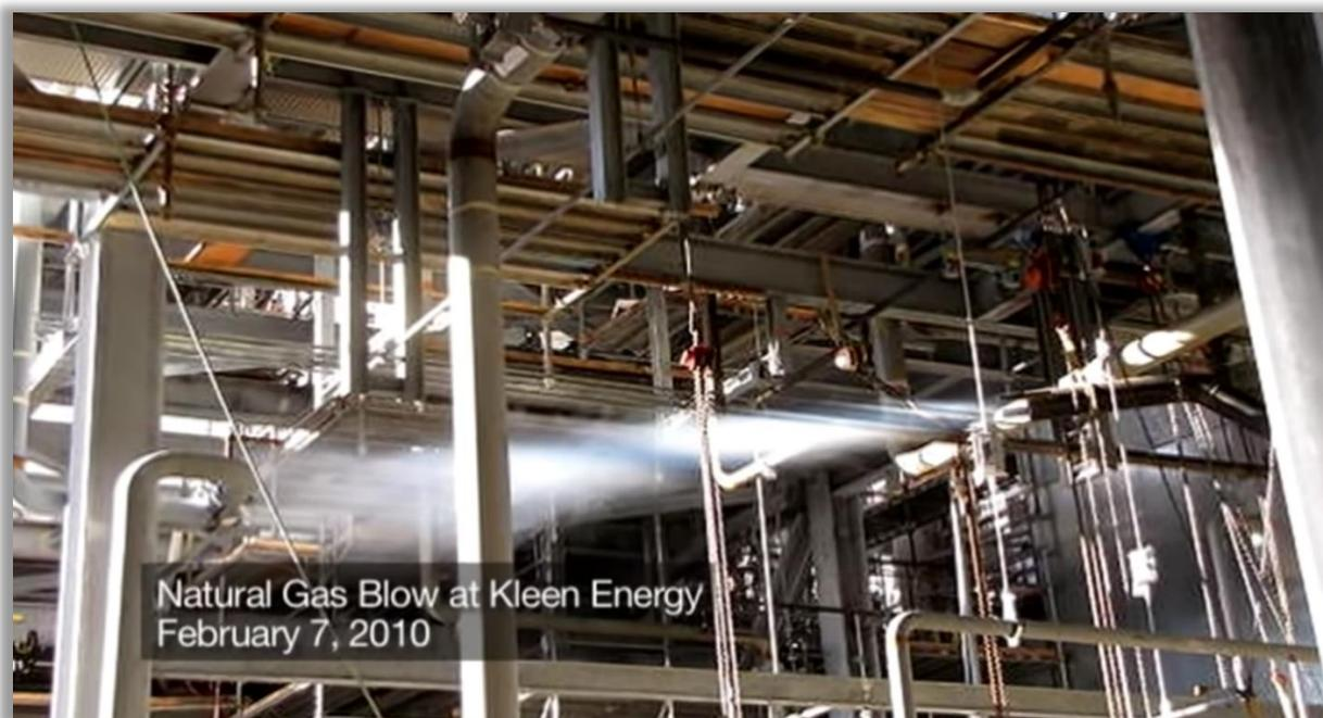
**Figure 28.** Horizontal Natural Gas Blow at Kleen Energy. (Credit: CSB [83])
