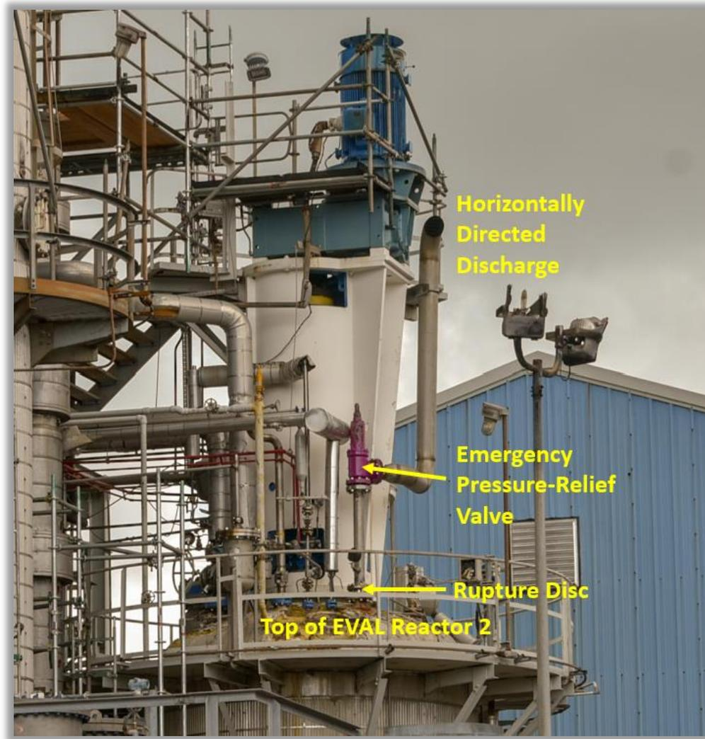
**Figure 7.** EVAL Reactor 2 Emergency Pressure-Relief System. (Credit: CSB)
