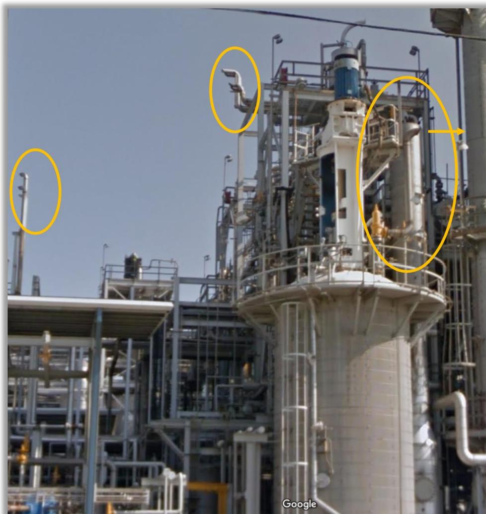
**Figure 19.** Horizontally Aimed Discharge Piping. (Credit: Google Maps annotated by CSB)
