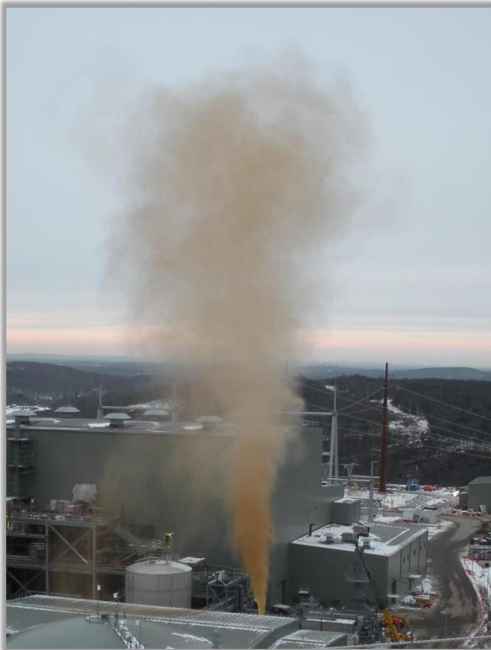
**Figure 30.** Vertical Natural Gas Blow at Kleen Energy.<sup>a</sup> (Credit: CSB [83])
