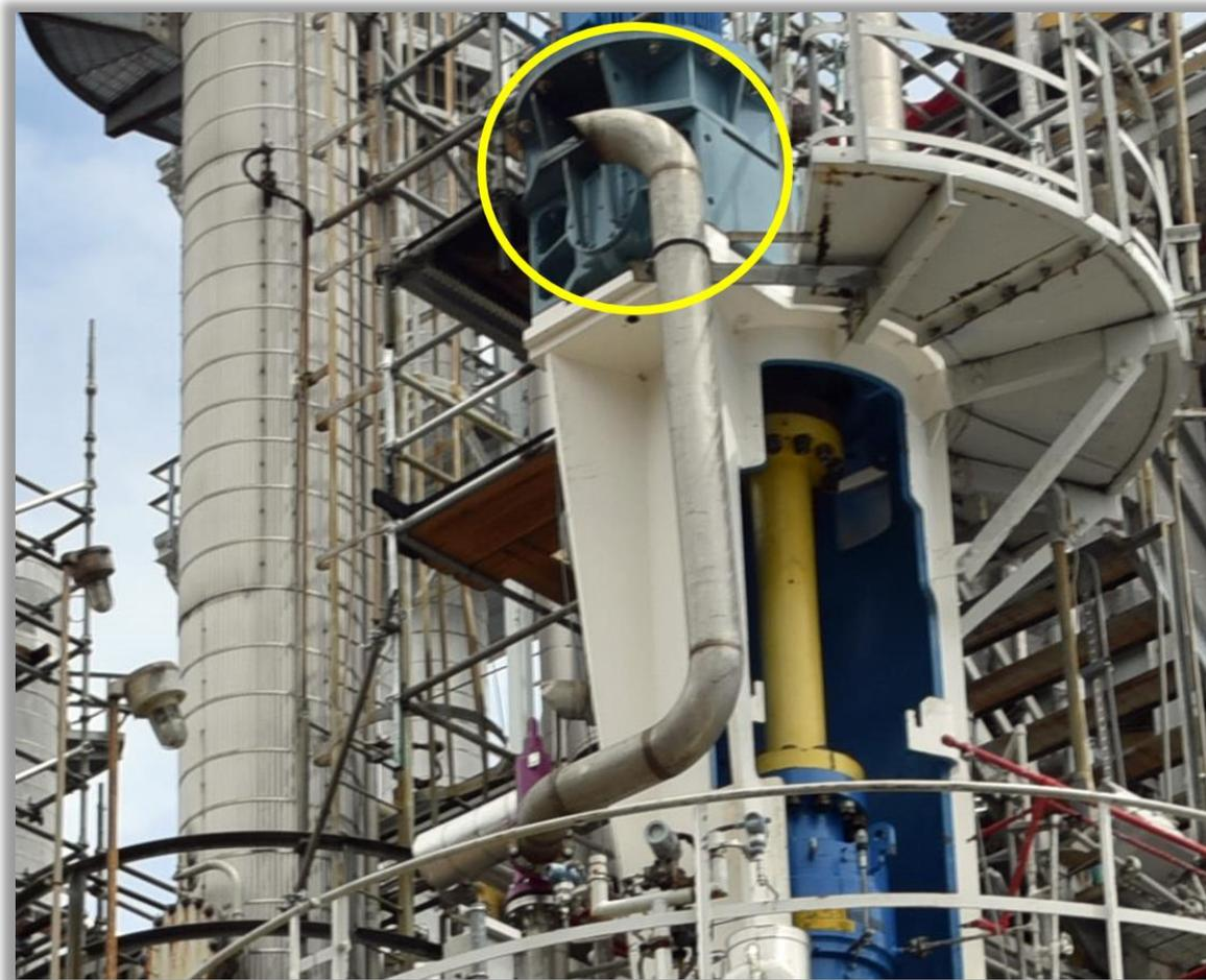
**Figure 8.** EVAL Reactor 2 Emergency Pressure-Relief System Outlet Piping. (Credit: CSB)
