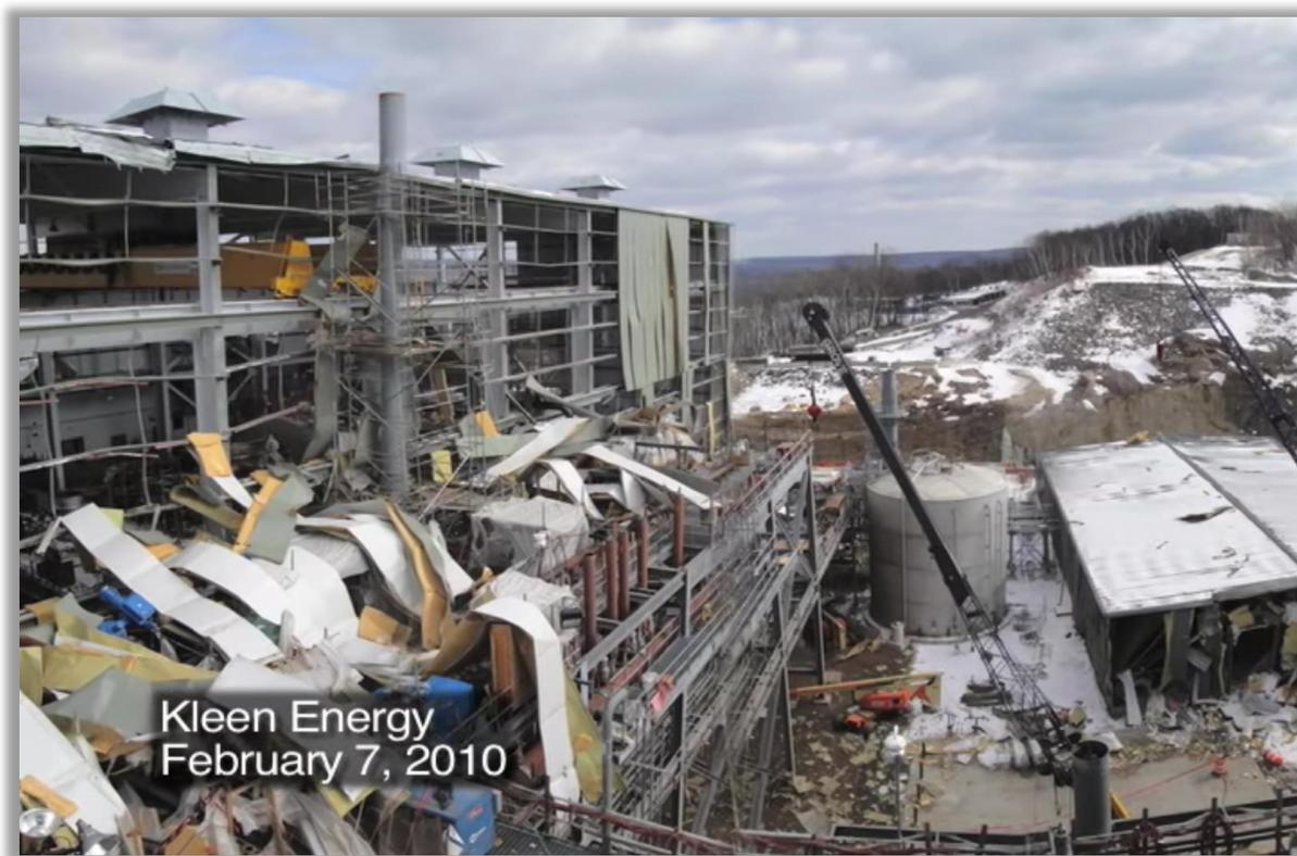
**Figure 29.** Explosion Damage at Kleen Energy. (Credit: CSB [84])
